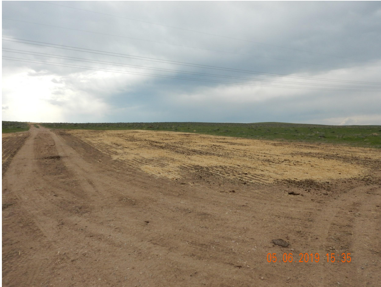
Photo 2. Photo taken from the southern tank battery location, facing South. See comments under Photo 1.
