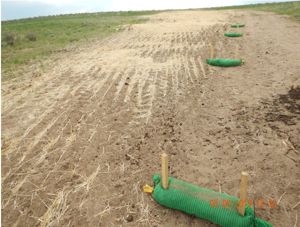
Photo 3. Photo taken from the former well location access road, facing West. Operator has repaired erosion along the access road and installed temporary BMPs in response to the previous corrective action inspection.
