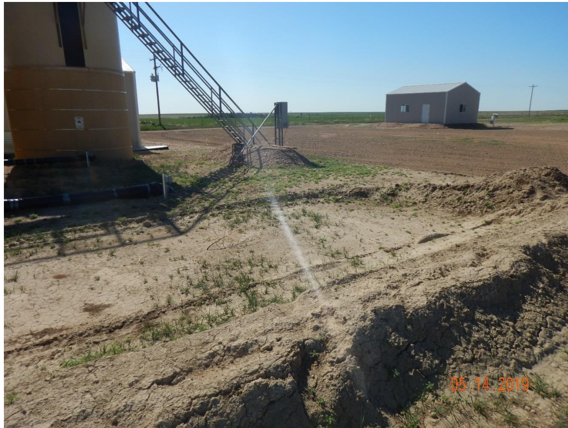
Photo 2: Photo taken from the tank battery, facing southeast. Photo shows secondary containment at battery remains insufficient.
