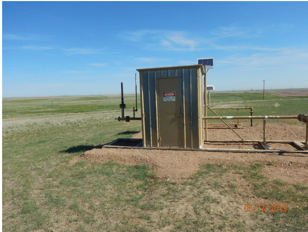
Photo 3: Photo taken from the west end of the location, facing north. Photo shows meter shed where gas is freely venting.
