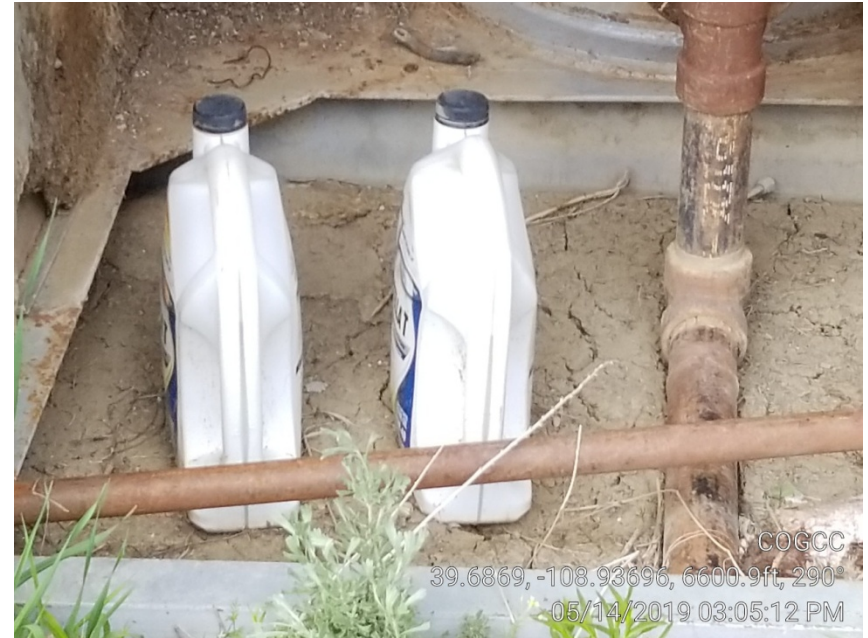
Photo 3. Motor oil stored in separator on ground without secondary containment.
