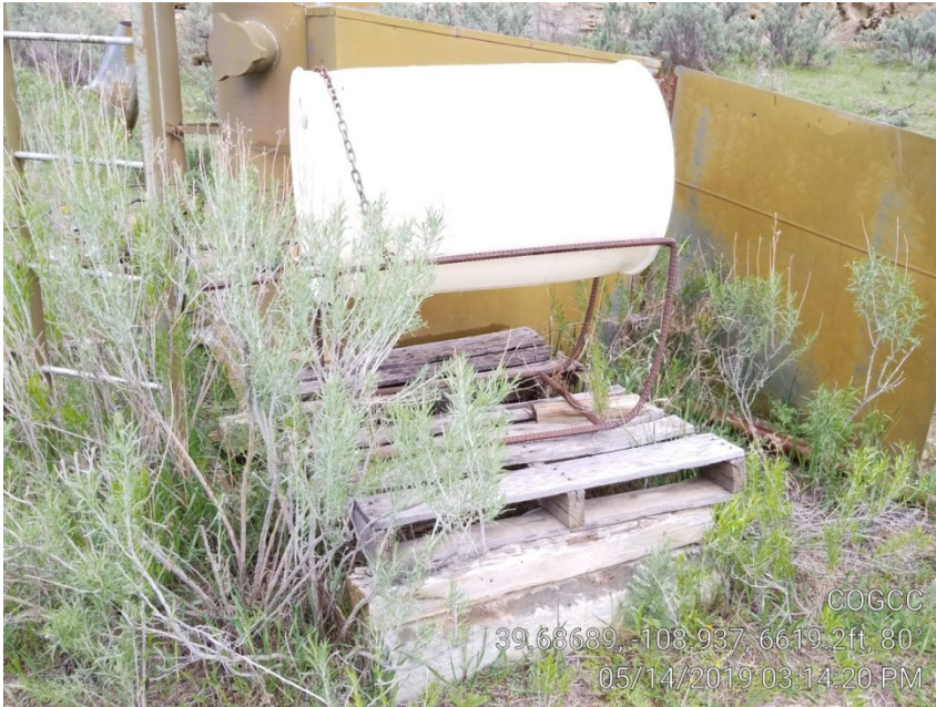
Photo 2. Empty container of corrosion inhibitor without secondary containment on pallets.
