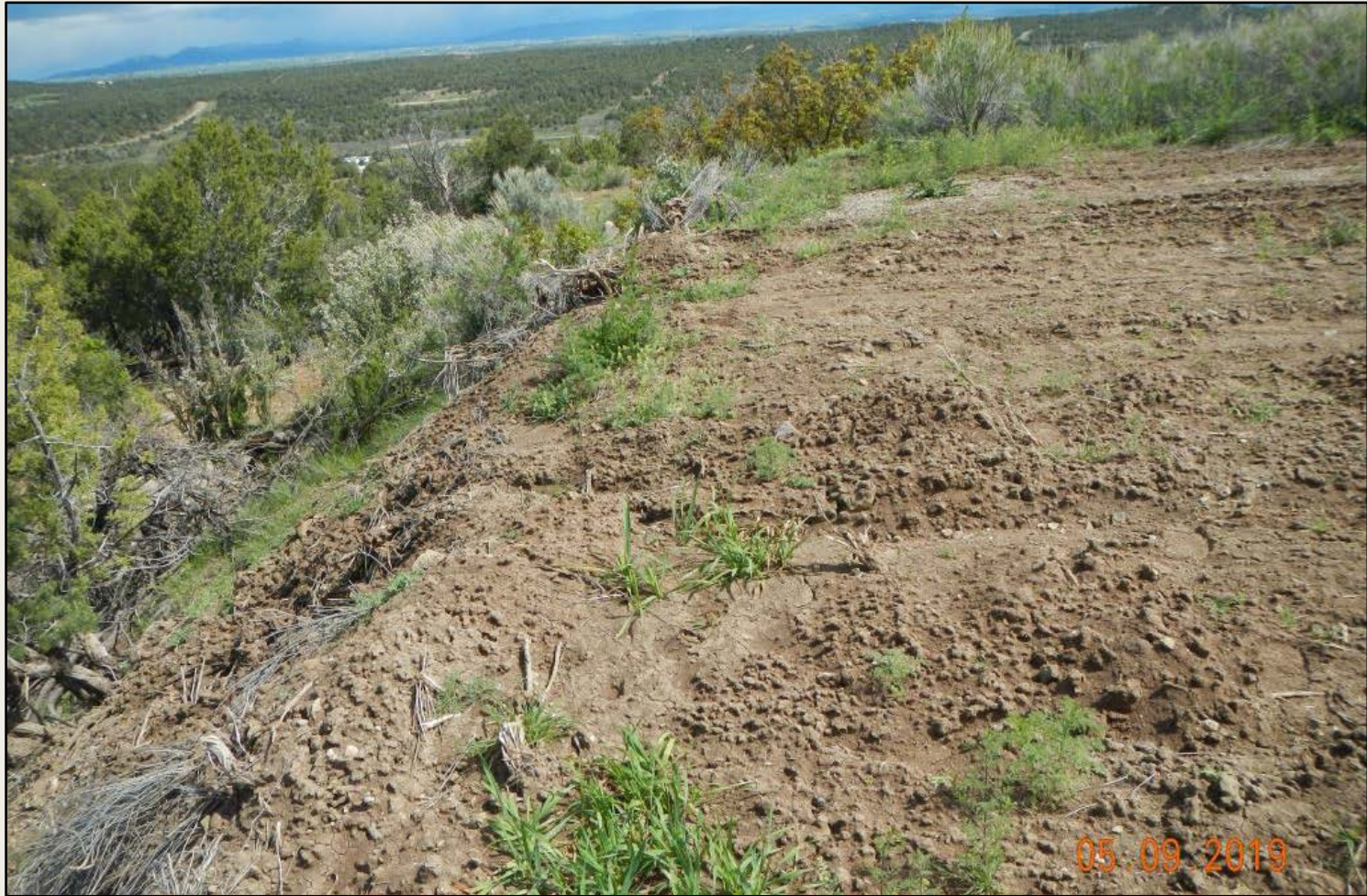
Photo 1. View of disturbance area in the western project area, needing stormwater controls and reclamation.
