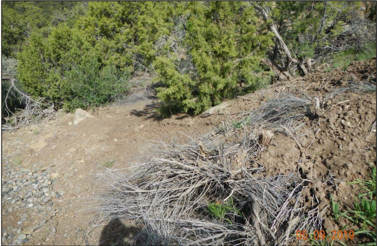
Photo 2. Downslope of disturbance area in the western project area where soil was pushed down-slope. Sediment controls are needed here.
