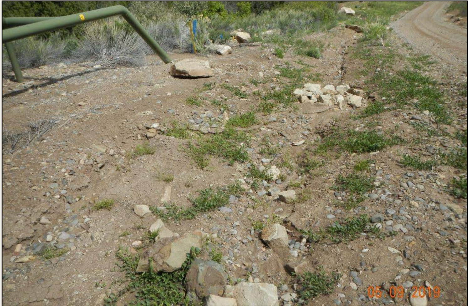
Photo 5. View of erosional channeling at the well pad entrance, and along the access road. BMPs are not sufficient in this area. Road was recently improved, appears to have been crowned, graveled, and ditched.
