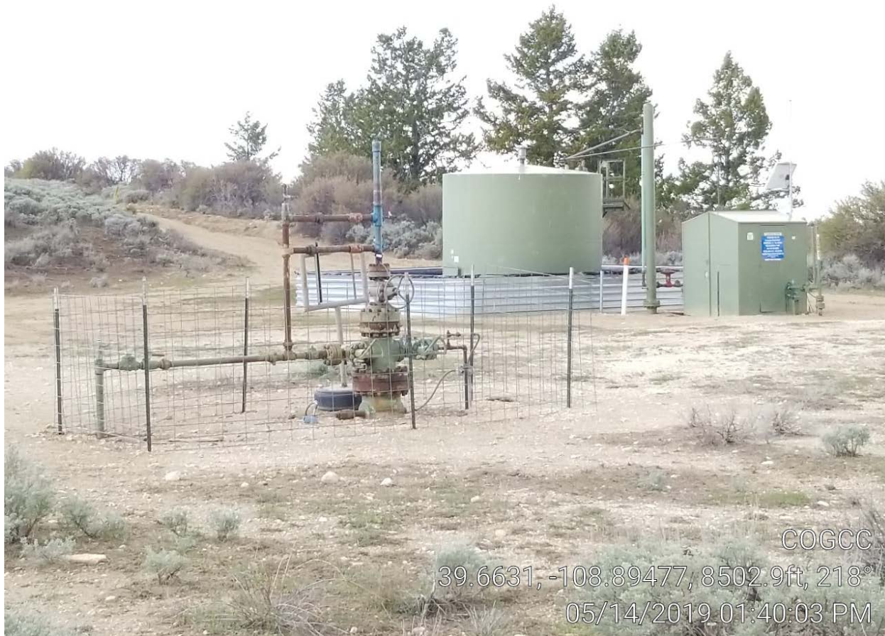
Photo 1. Location looking southwest.
