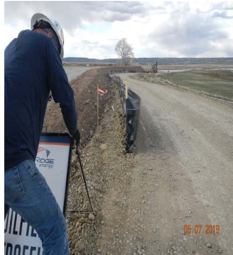
Photo#3: Silt fence is installed around perimeter of Location expansion.
