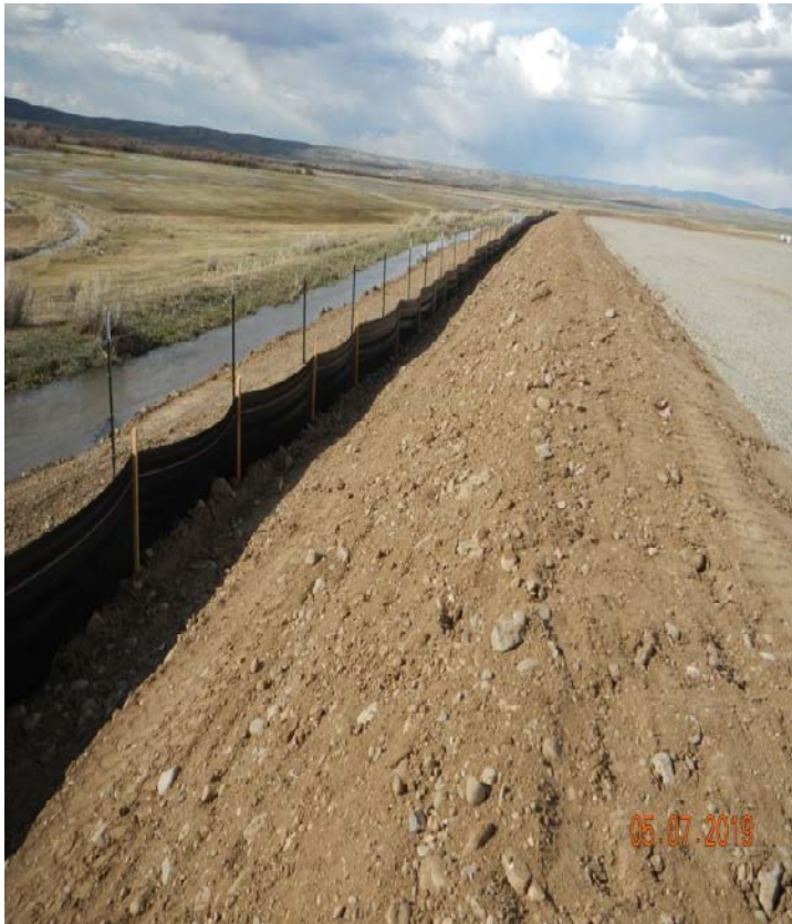
Photo#2: Silt fence is installed around perimeter of Location expansion.
