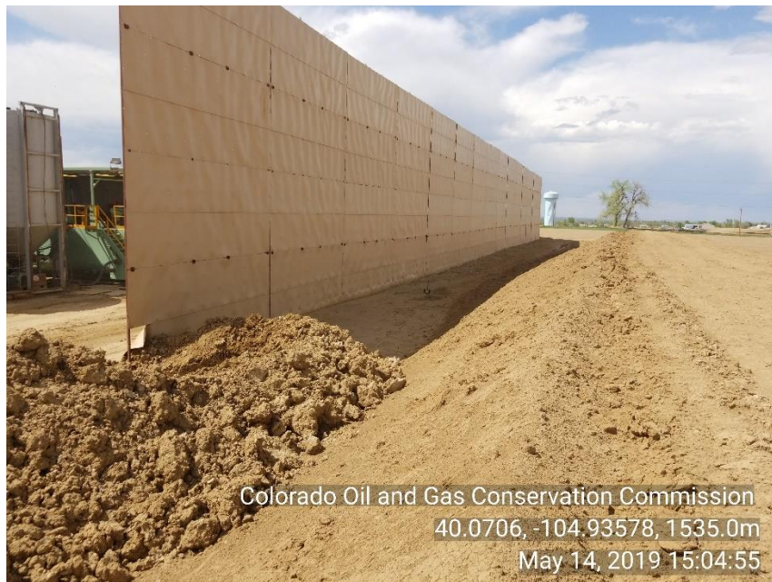
Photo 5 Protection of soils and storm water: material being pushed up on top soil pile and also blocking drainage ditch of location. Sediment building up behind pushed up material possible storm water issue.
