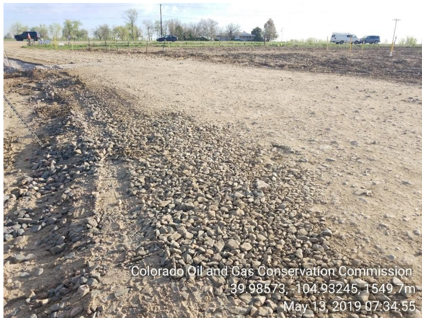
Photo 15 Tracking pad: Rock tracking pad impacted with sediment not properly maintained.
