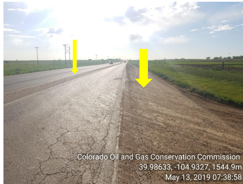
Photo 20 Vehicle tracking: Sediment from access road being carried onto HWY 7 .
