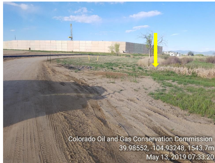
Photo 14 Storm water: no BMP's in place to control sediment from leaving access road to location. Sediment is running off and covering vegetation.
