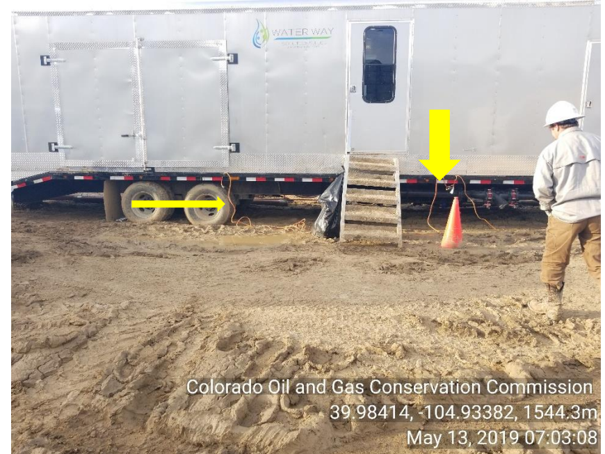
Photo 2 electric cords laying in mud and water.
