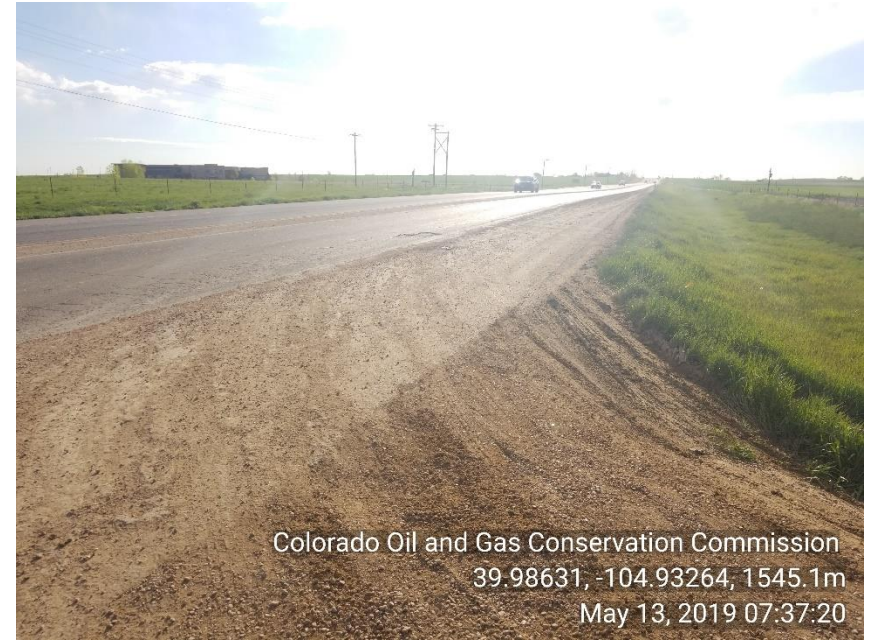
Photo 18 Vehicle tracking: Sediment from access road being carried onto HWY 7 .
