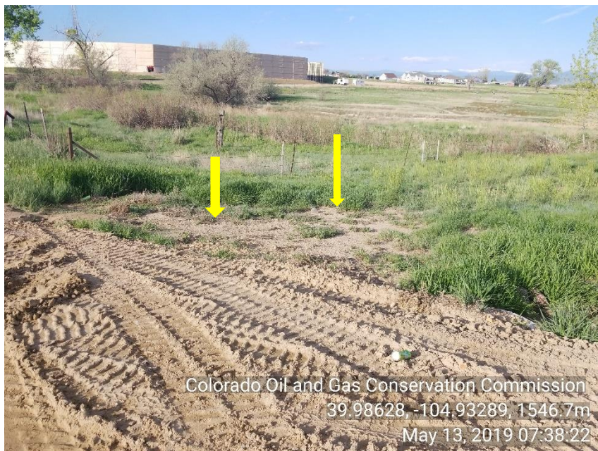
Photo 21 Storm water Improper BMP's sediment being carried off access road into vegetation.
