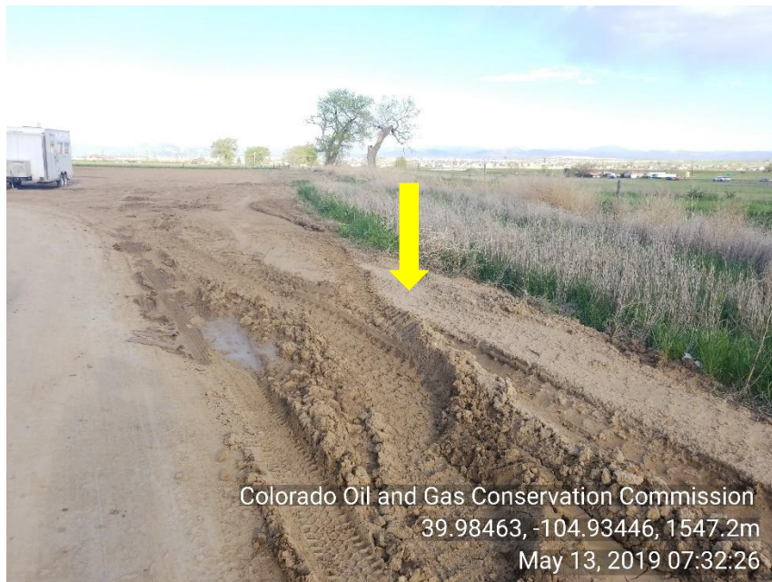
Photo 13 Build up of mud and water improper drainage and no BMP's in place to control sediment from leaving access road to location.
