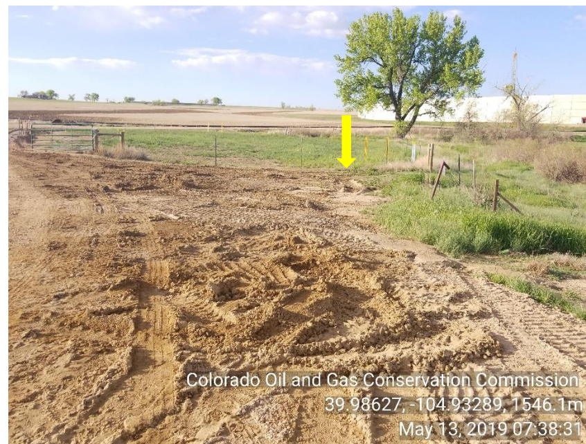
Photo 22 Storm water Improper BMP's sediment being carried off access road into vegetation.
