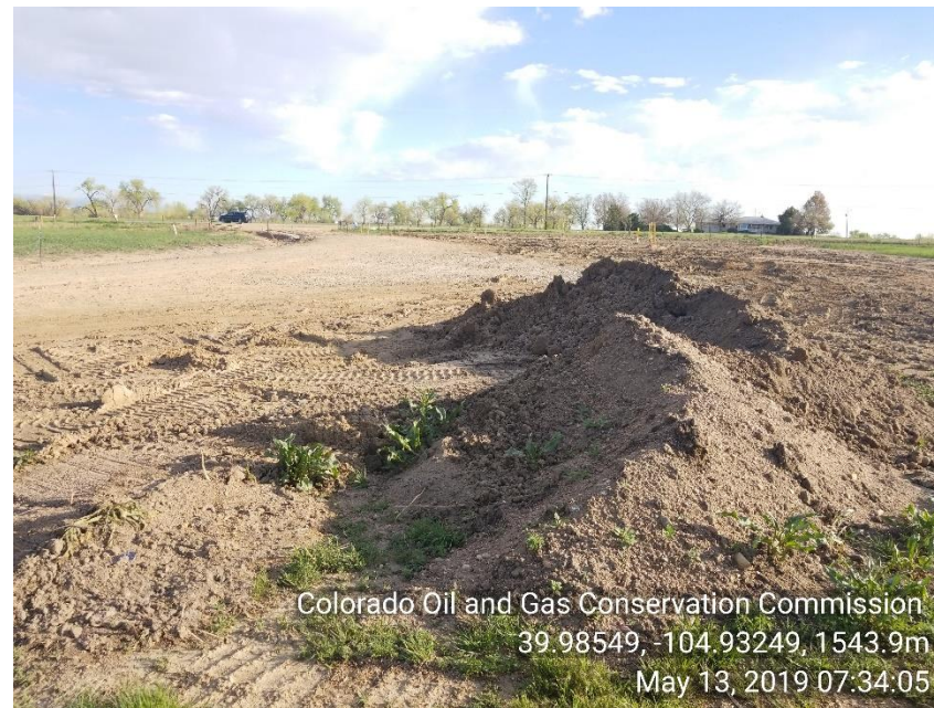
Photo 16 Storm water: no BMP's in place to control sediment from leaving access road to location.
