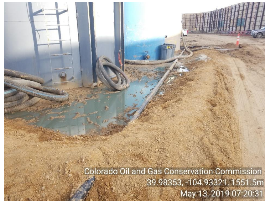
Photo 8 Spill release: unknown fluid in drill out tank containment.
