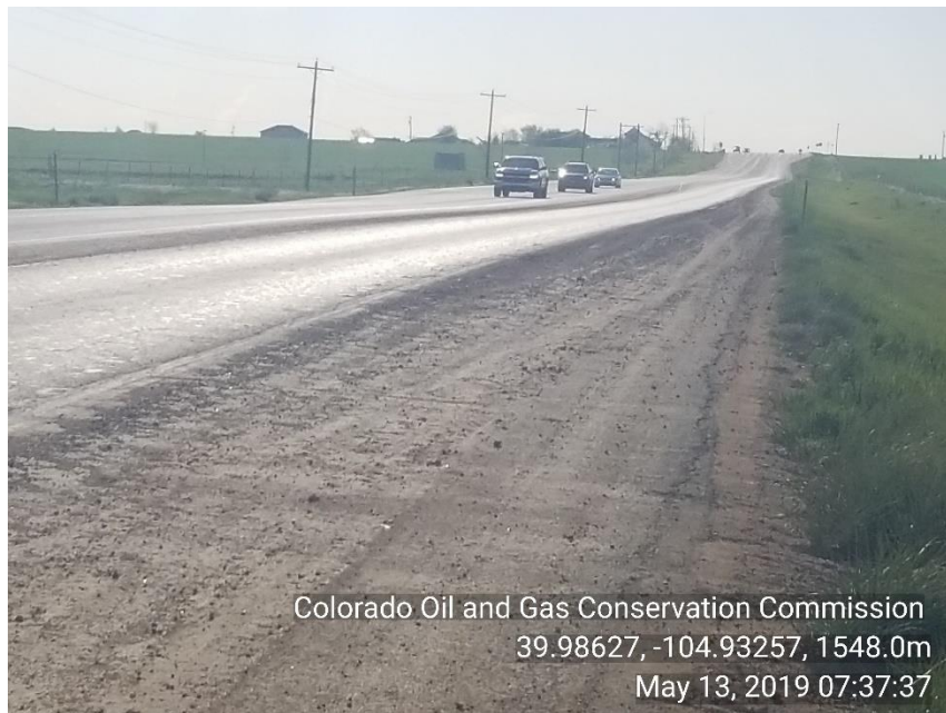
Photo 19 Vehicle tracking: Sediment from access road being carried onto HWY 7 .
