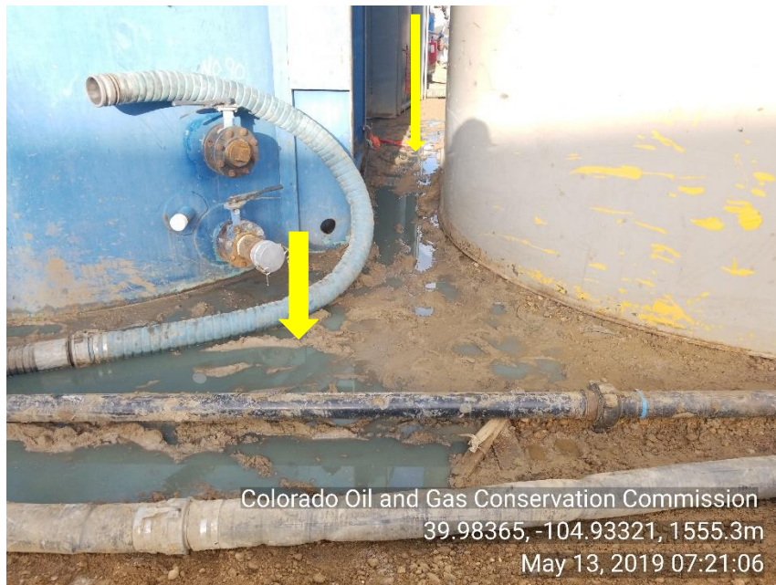
Photo 11 Spill release: unknown fluid in drill out tank containment.
