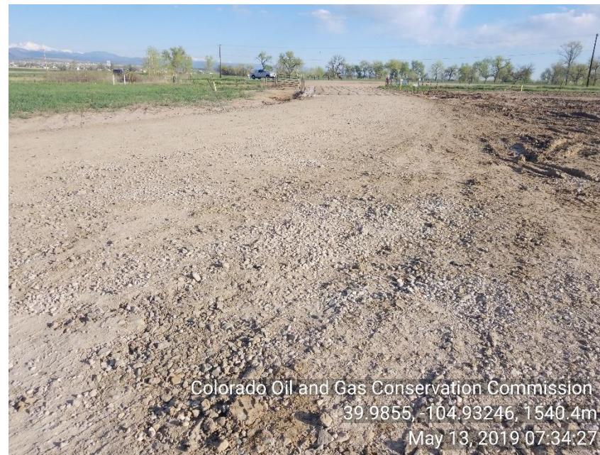
Photo 16 Tracking pad: Rock tracking pad impacted with sediment not properly maintained.
