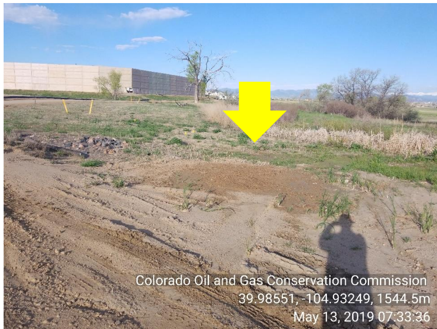
Photo 15 Storm water: no BMP's in place to control sediment from leaving access road to location. Sediment is running off and covering vegetation.
