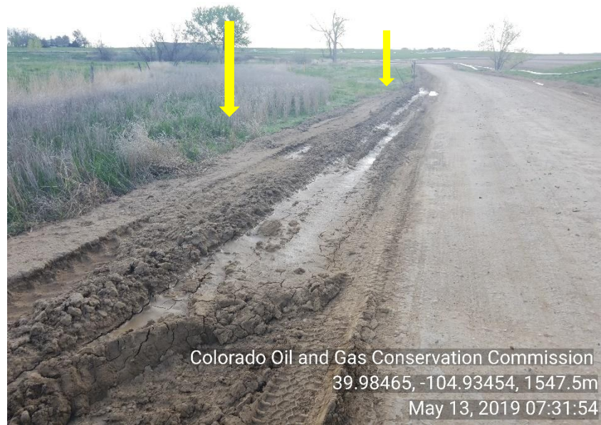
Photo 12 Build up of mud and water improper drainage and no BMP's in place to control sediment from leaving access road to location.
