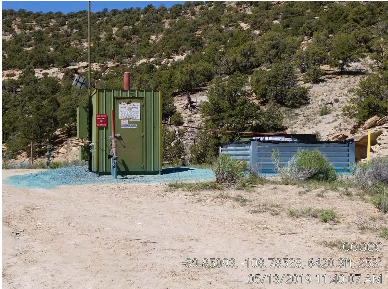
Photo 1. Location looking west.
