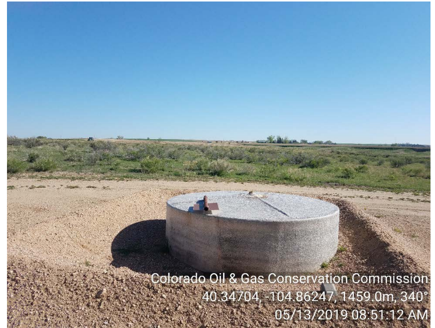
Produced water vault at separator
