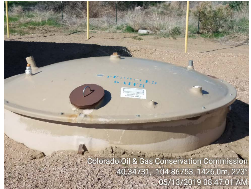
Produced water vault at tank battery
