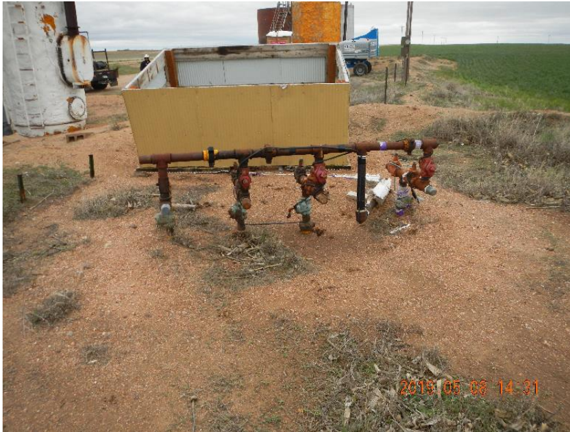
Photo 3: Valve manifold with metal shed upside down in the background.
