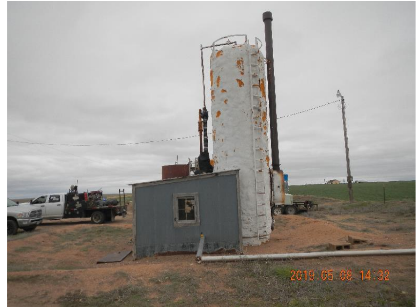
Photo 4: Vertical heated separator with metal shed.
