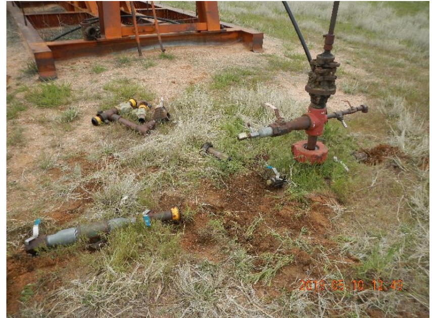
Photo 8: Wellhead with flow line disconnected and valves plugged.
