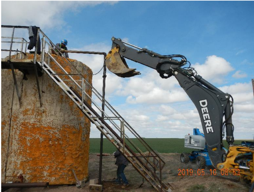
Photo 7: Disconnecting flow line from separator.
