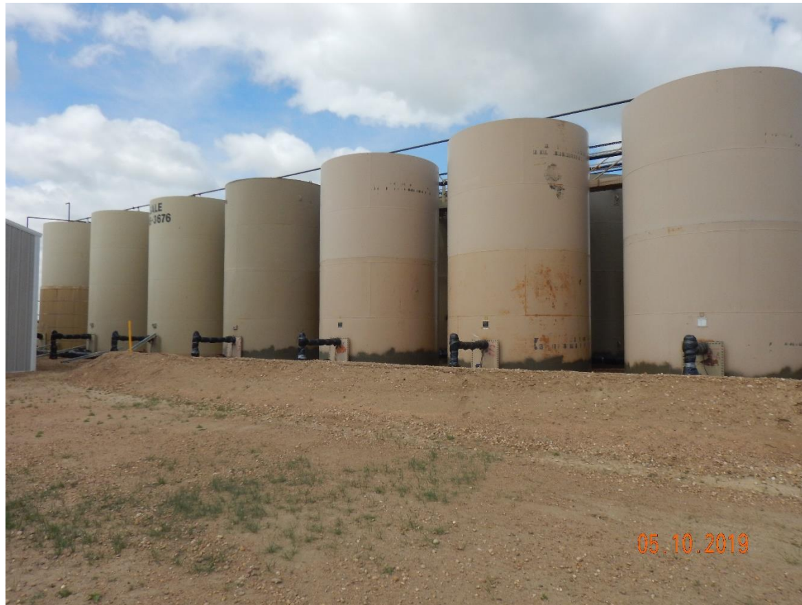
Photo 1: Photo taken from the northeast end of the tank battery, facing southwest. Photo shows insufficient signage/labeling on tanks in accordance with 210.d
