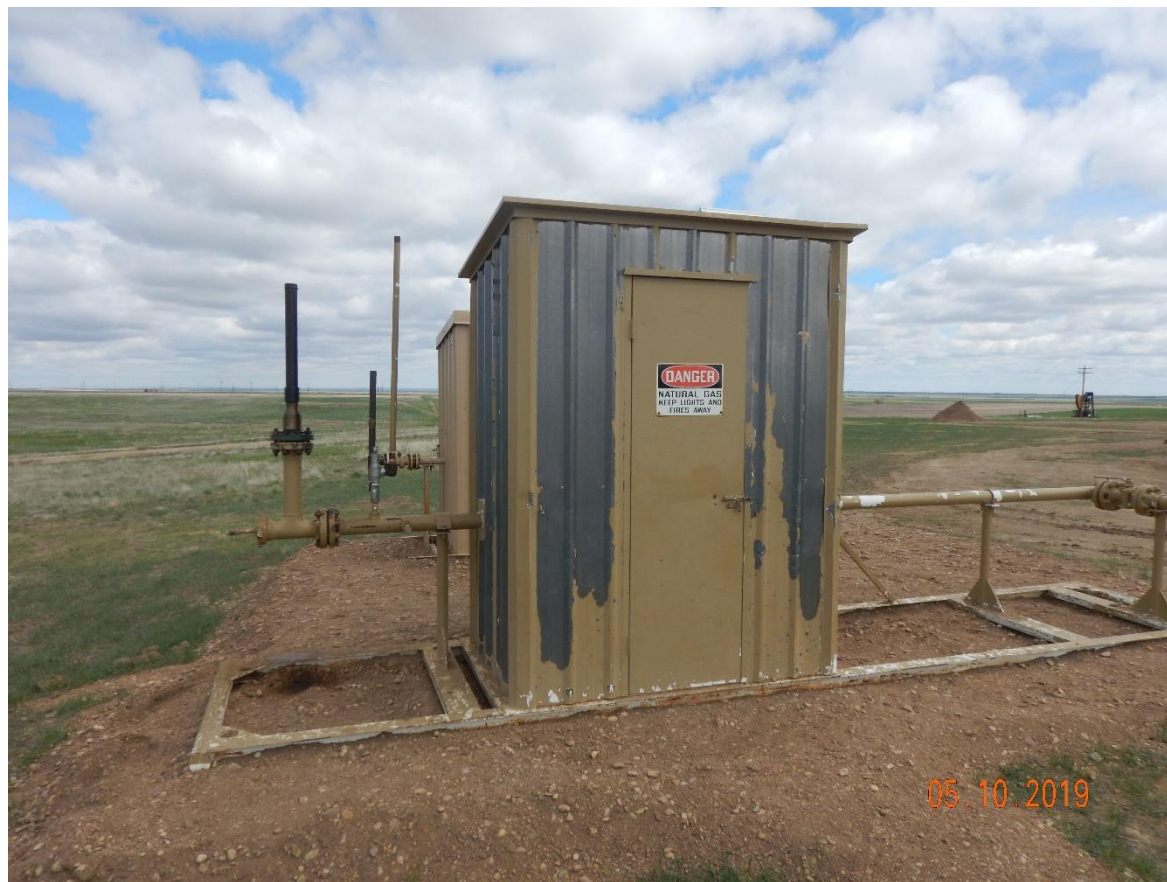
Photo 6: Photo taken from the west end of the location. Photo of shows meter run. Inspector audibly detected what appear to be gas freely venting from meter run. Inspector confirmed with PCR that gas venting was being conducted.
