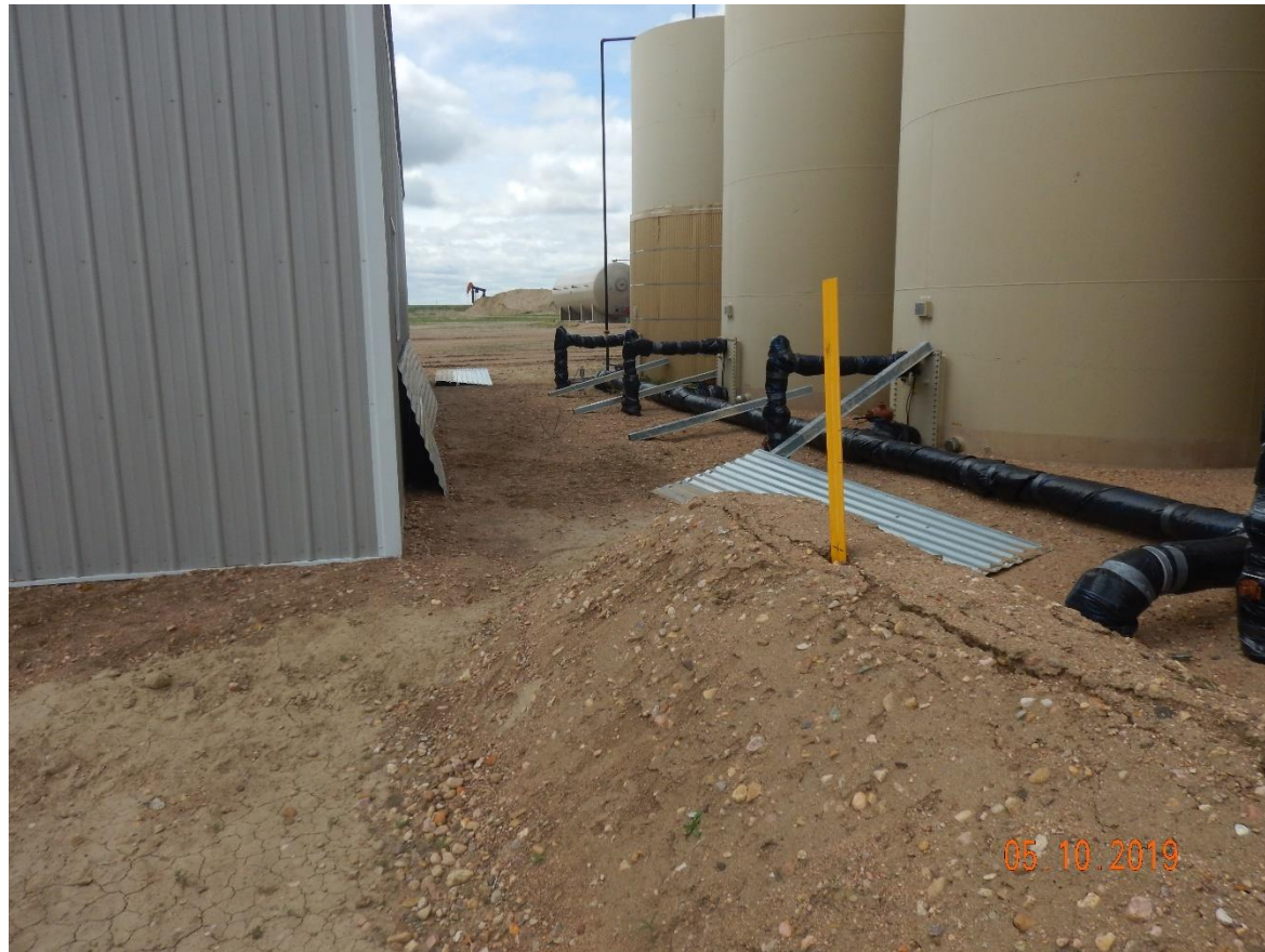
Photo 2: Photo taken from the east end of the tank battery, facing south. Photo shows insufficient secondary containment at tanks.
