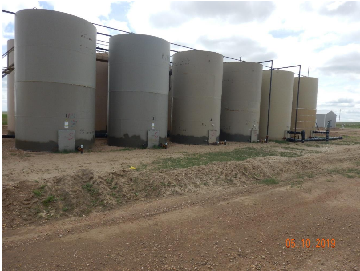
Photo 3: Photo taken from the west end of the tank battery, facing southeast. Photo shows insufficient secondary containment at tanks. Photo shows insufficient signage/labeling on tanks in accordance with 210.d. Photo also shows insufficient secondary containment at tanks.
