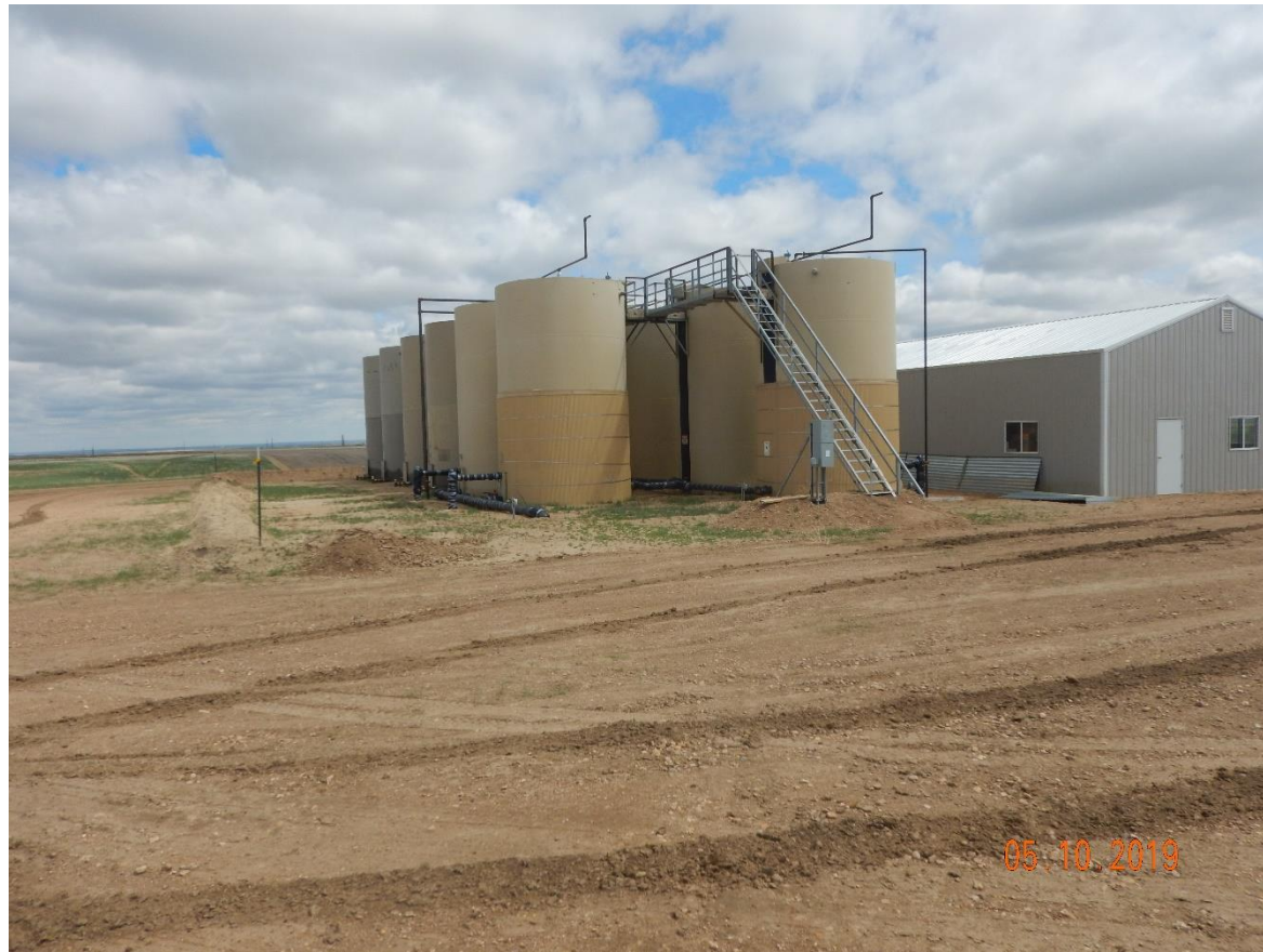
Photo 4: Photo taken from the south end of the tank battery, facing northeast. Photo shows insufficient secondary containment at tanks. Photo shows insufficient signage/labeling on tanks in accordance with 210.d. Photo also shows insufficient secondary containment at tanks.
