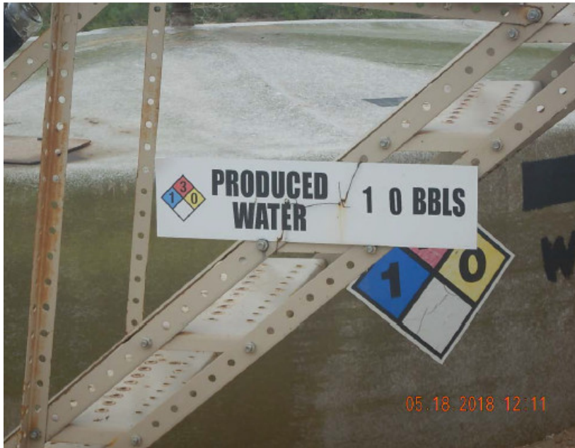
Photo #5 Cache 17-52, 17-21 Battery Produced H2O vault– Incorrect Capacity posted from prior FIR
