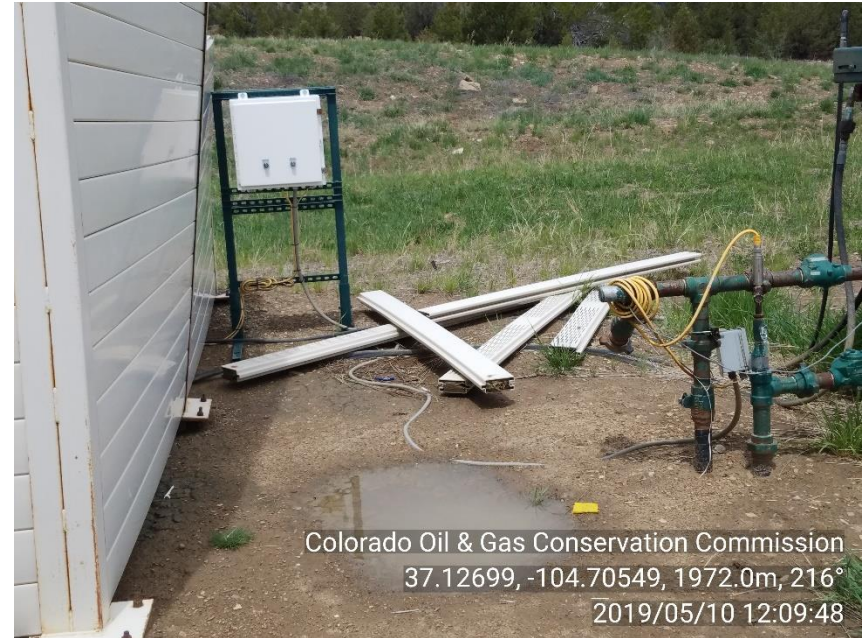
PHOTO 6: UNUSED EQUIPMENT/ SOUND WALLS IN DISREPAIR. COMPLY WITH RULE 603.f. REPAIR SOUND WALLS. CA DATE 6/10/19
