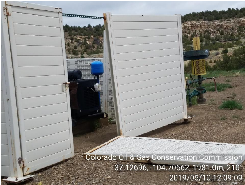
PHOTO 3: UNUSED EQUIPMENT/ SOUND WALLS IN DISREPAIR. COMPLY WITH RULE 603.f. REPAIR SOUND WALLS. CA DATE 6/10/19
