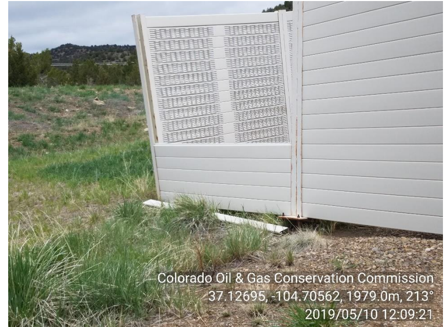
PHOTO 4: UNUSED EQUIPMENT/ SOUND WALLS IN DISREPAIR. COMPLY WITH RULE 603.f. REPAIR SOUND WALLS. CA DATE 6/10/19
