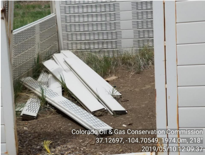
PHOTO 5: UNUSED EQUIPMENT/ SOUND WALLS IN DISREPAIR. COMPLY WITH RULE 603.f. REPAIR SOUND WALLS. CA DATE 6/10/19
