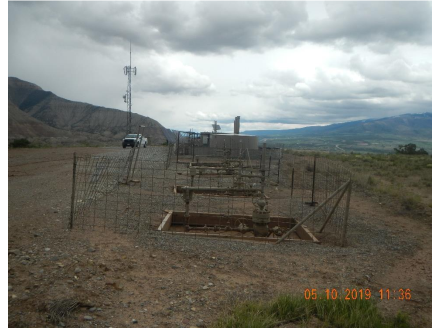
Fence has been repaired.
