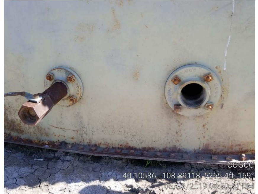
Photo 7. Tank 2 open port.
