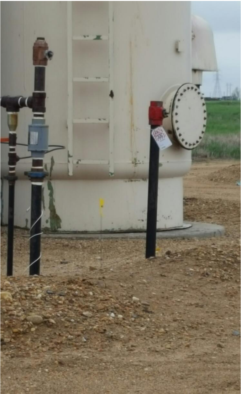
Figure #1 Deadman and riser have been marked.
