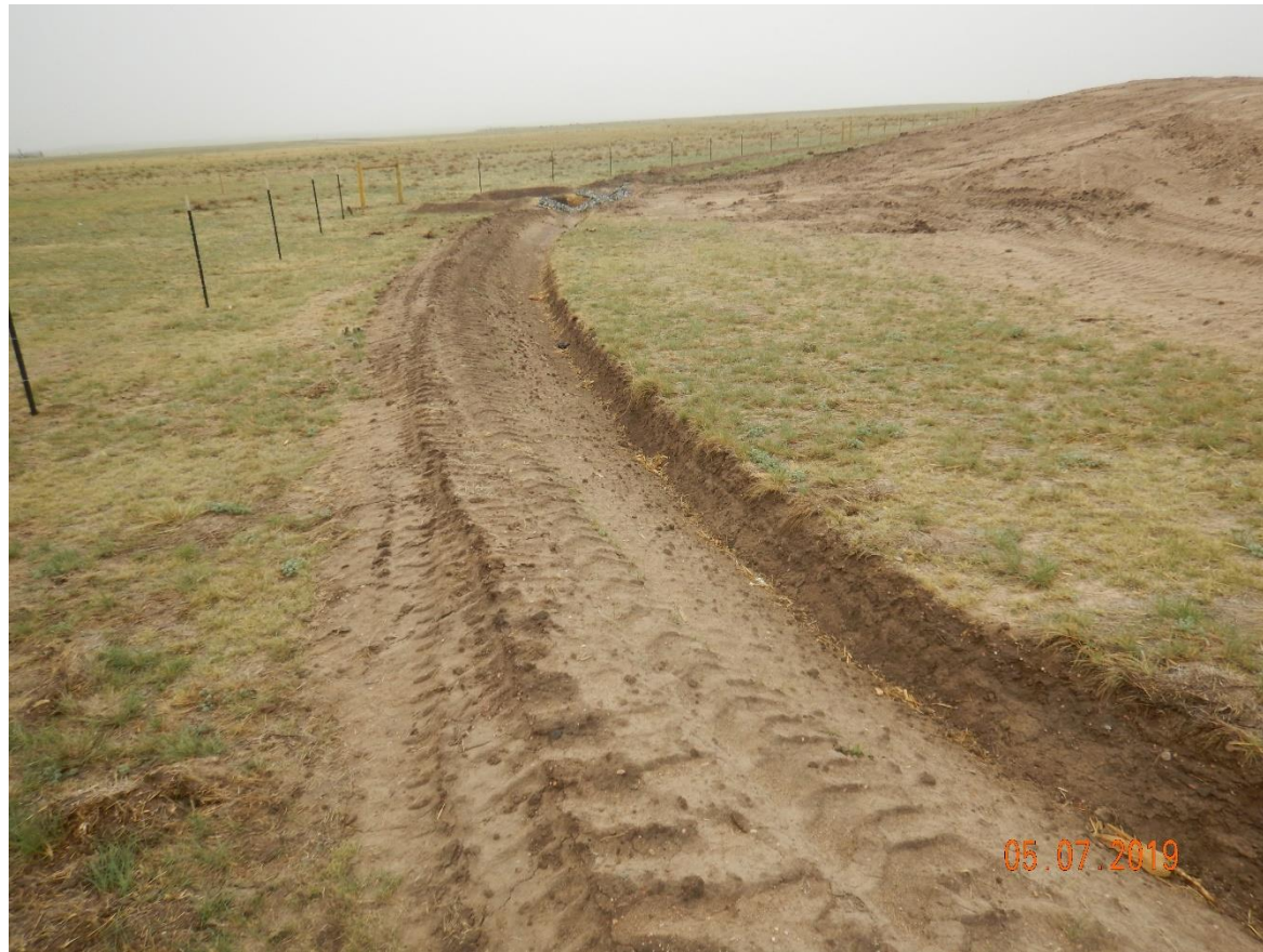
Photo 11: Photo taken from the southeast corner of the location, facing southwest. Photo shows stormwater ditch along perimeter of location. See comments under photo 10
