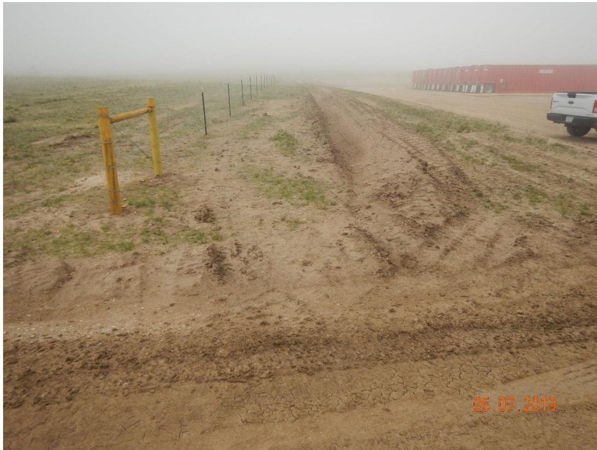
Photo 16: Photo taken from the west end of the location. Photo shows area where the ditch abruptly ends without sufficient outlet protection to allow for sediment laden free stormwater discharge; ditch has not been constructed in accordance with good engineering practices.
