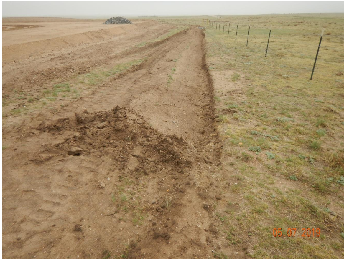
Photo 5: Photo taken from the wet end of the location, facing south. Photo shows stormwater ditch along perimeter of location. BMP appears to have been constructed with a blade leaving a vertical grade of unconsolidated material. Ditch has not been constructed in accordance with good engineering practices.
