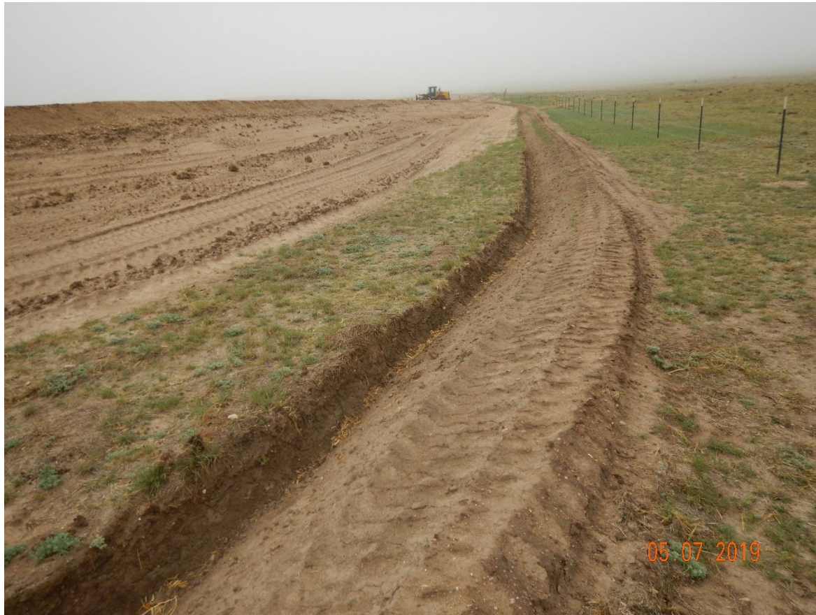
Photo 10: Photo taken from the southeast corner of the location, facing north. Photo shows stormwater ditch along perimeter of location. BMP appears to have been constructed with a blade leaving a vertical grade of unconsolidated material. Ditch has not been constructed in accordance with good engineering practices.
