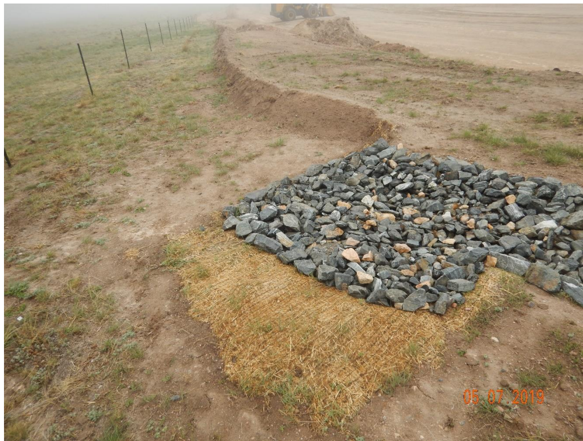
Photo 17: Photo taken from the northeast corner of the location. Photo shows outlet that appears to be sufficiently armored to allow for sediment laden free stormwater discharge from the northeast end of the location.
