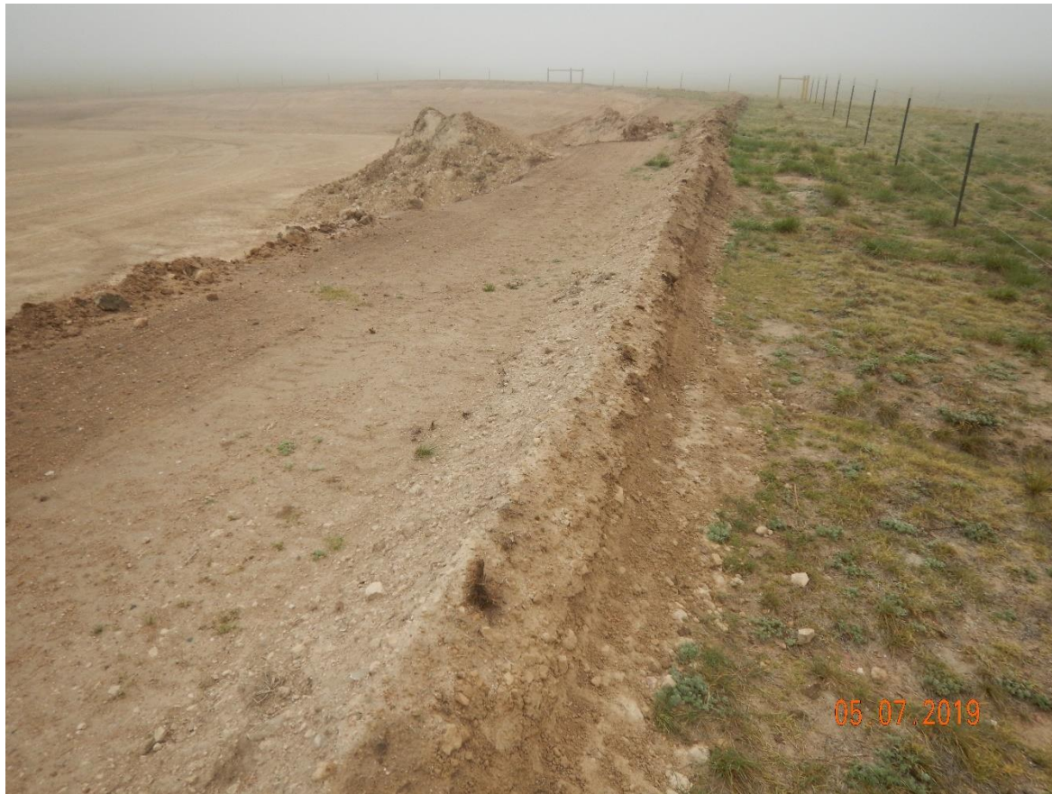
Photo 14: Photo taken from the northeast end of the location, facing north. Photo shows areas where operator installed a berm along perimeter of the location. Berms have not been consolidated in accordance with good engineering practices. Berms remain loose material and a potential pollutant source.
