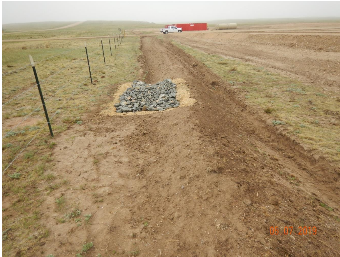
Photo 6: Photo taken from the southwest end o the location, facing north. Photo shows outlet armoring at the stormwater ditch.
