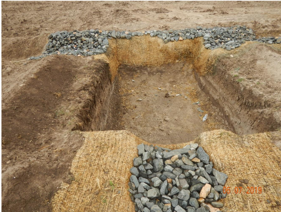
Photo 8: Photo taken from the southeast corner of the location. Photo of sediment trap. Operator has installed one (1) sediment trap on the southeast end of the location. Sediment trap does not appear to be sufficient in size to manage stormwater runoff from the 8.26 acre pad. Additionally, sediment has been constructed with vertical slopes rather than a grade, that will likely promote erosion degradation within the BMP. Sediment trap does not appear to have been constructed in accordance with good engineering practices
