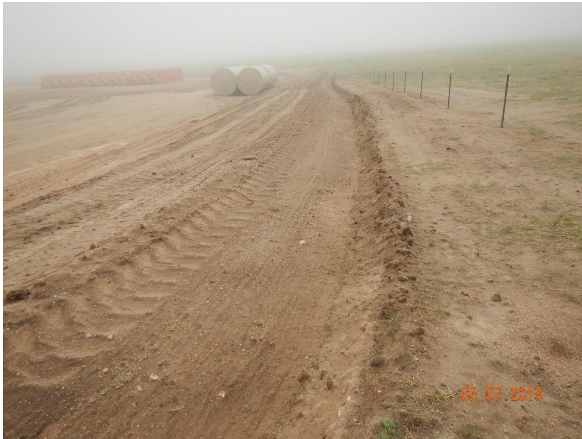
Photo 18: Photo taken from the northeast corner of the location, facing west. Photo shows ditch and berm along perimeter. Ditch to have been constructed with a blade leaving a vertical grade of unconsolidated material. Ditch has not been constructed in accordance with good engineering practices.
