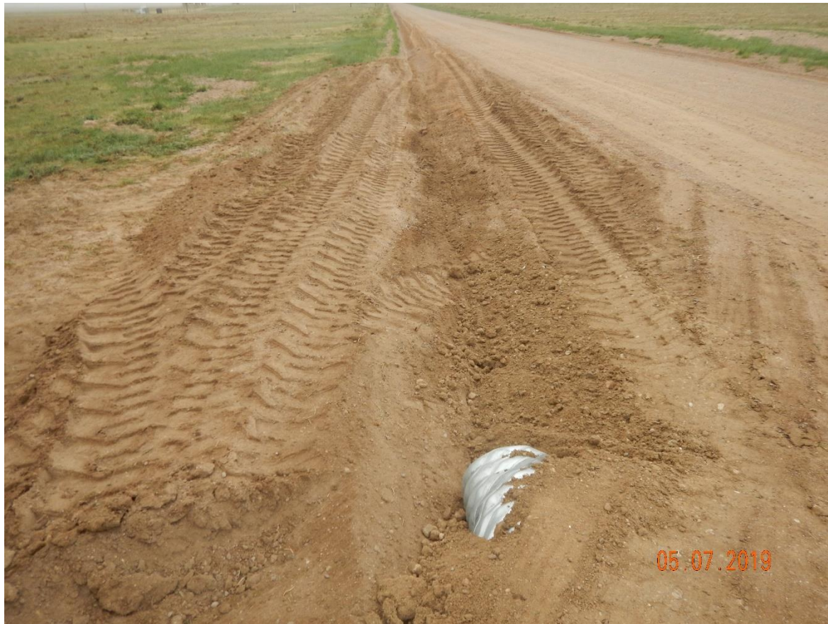
Photo 5: Photo of culvert at access road entrance.
