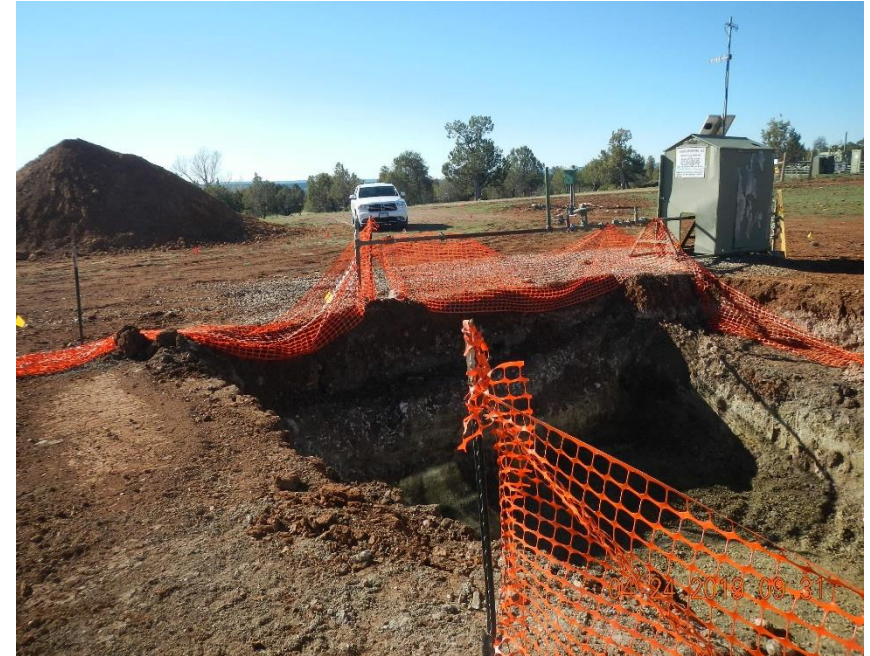
Excavation awaiting confirmation sample results prior to backfilling with stock piled fill dirt.
