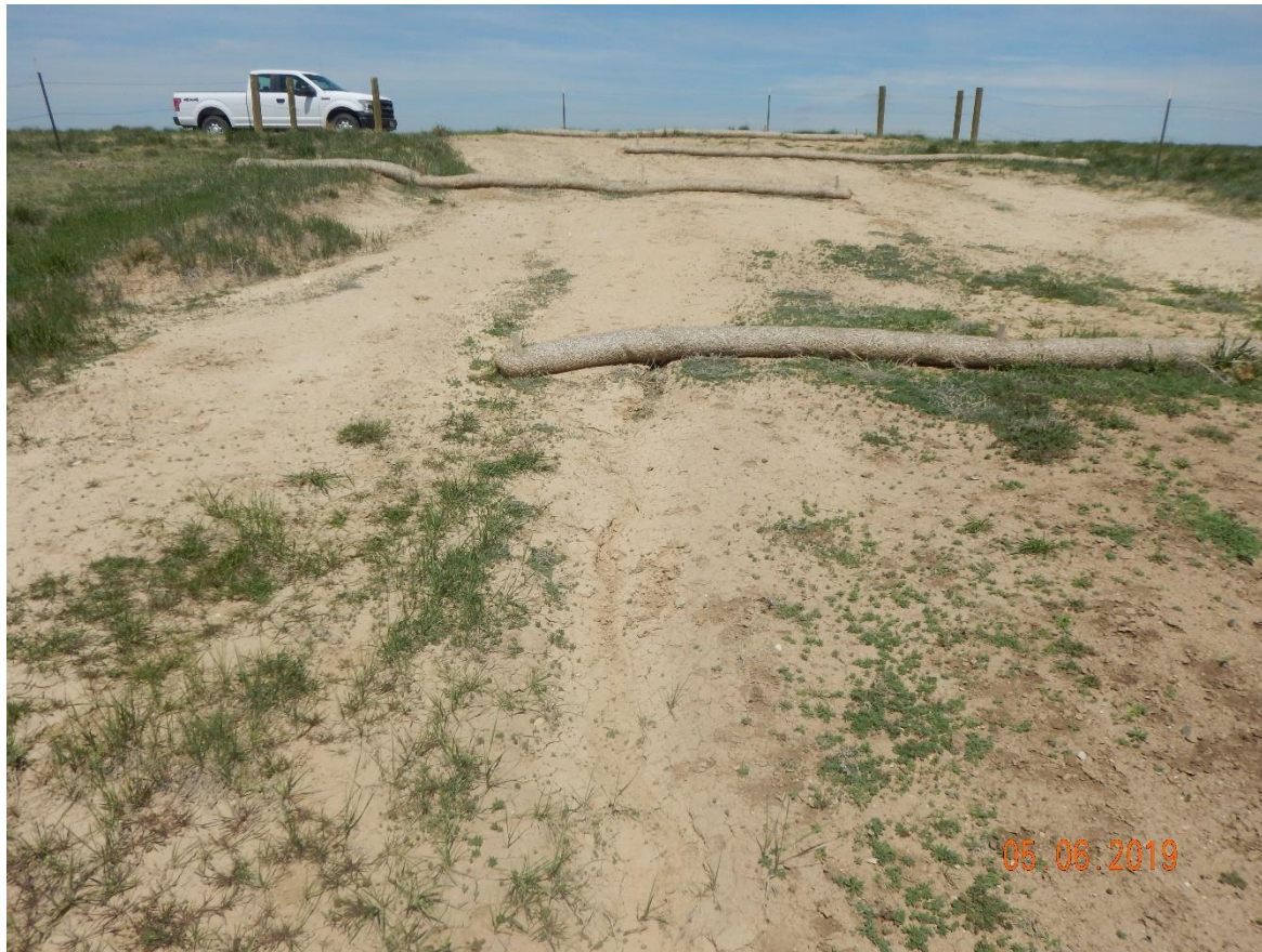
Photo 5: Photo taken from the location, facing north. Photo shows straw wattle BMPs are not in proper functioning condition, and are insufficient. Photo also shows the erosion degradation on the location.
