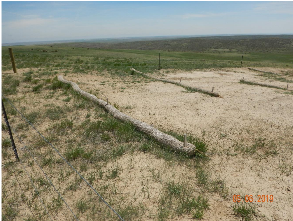
Photo 1: Photo taken from the northwest end of the location, facing east. Photo shows that location remains predominantly bare and exposed soil. Straw wattle BMPs remain insufficient and have not been installed in accordance with good engineering practices. No additional reclamation or stormwater management appears to have been conducted per corrective actions.
