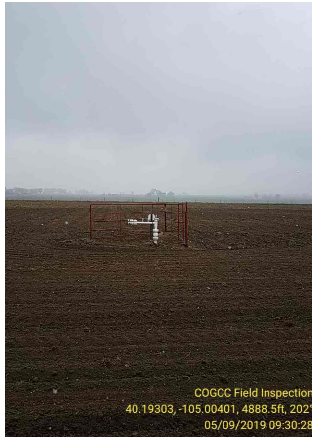
Photo 1 Gathering System Riser Remaining at Former Battery Location.
