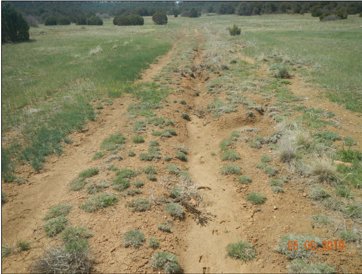
Photo 1. There is an erosion channel along the access road near the location.
