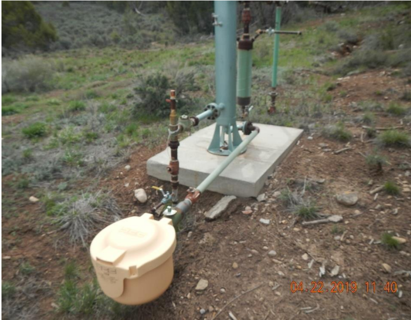
Drip pot on drop out tank.
