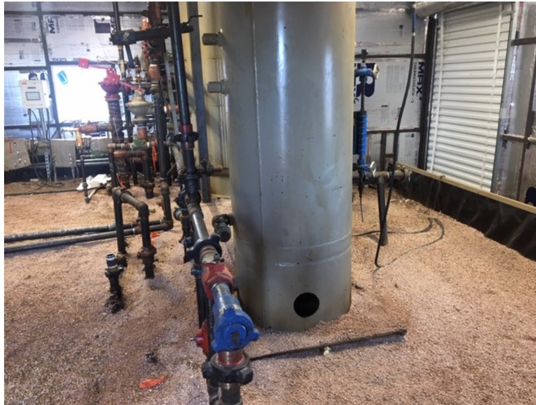
Photo 6 – Motu East Location ID 43945 Leaks within treater building reclaimed Corresponds with photo 4&5 of 4/15/2019 inspection
