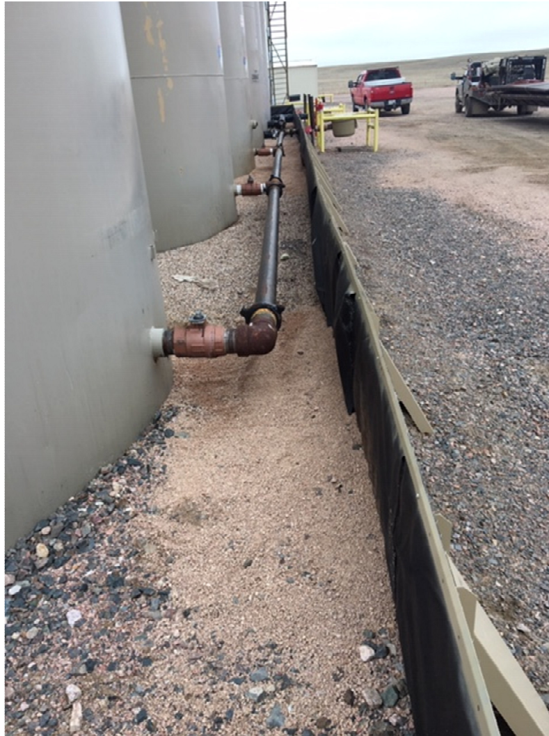
Photo 2 – Motu East Location ID 439459 Crude oil liquid load out line reclaimed
