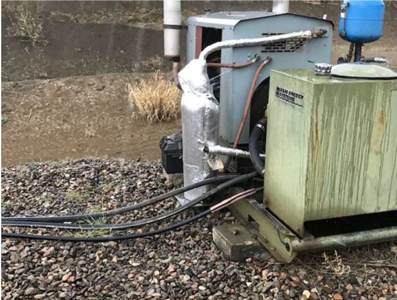
PHOTO 2: (PHOTO WAS TAKEN DURING RAIN SHOWERS) THE IMPACTED SOIL NEXT TO THE ENGINE SKID WAS REMOVED FROM THE LOCATION.
