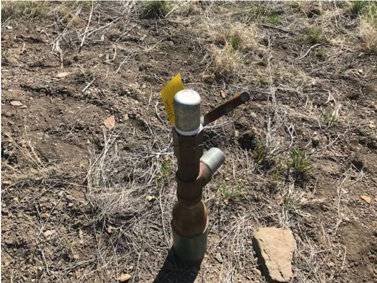
PHOTO 1: A BULL PLUG WAS INSTALLED ON THE RISER AND MARKED.
