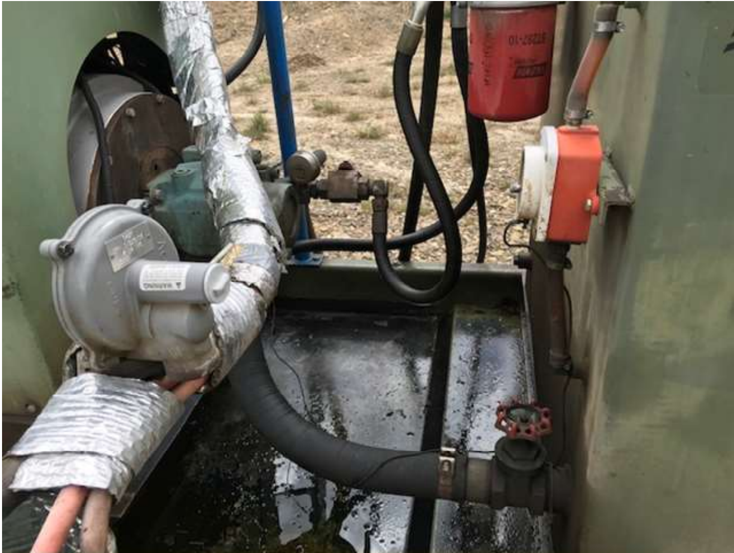
PHOTO 3: THE OIL ACCUMULATION IN THE CONTAINMENT WAS REMOVED.
