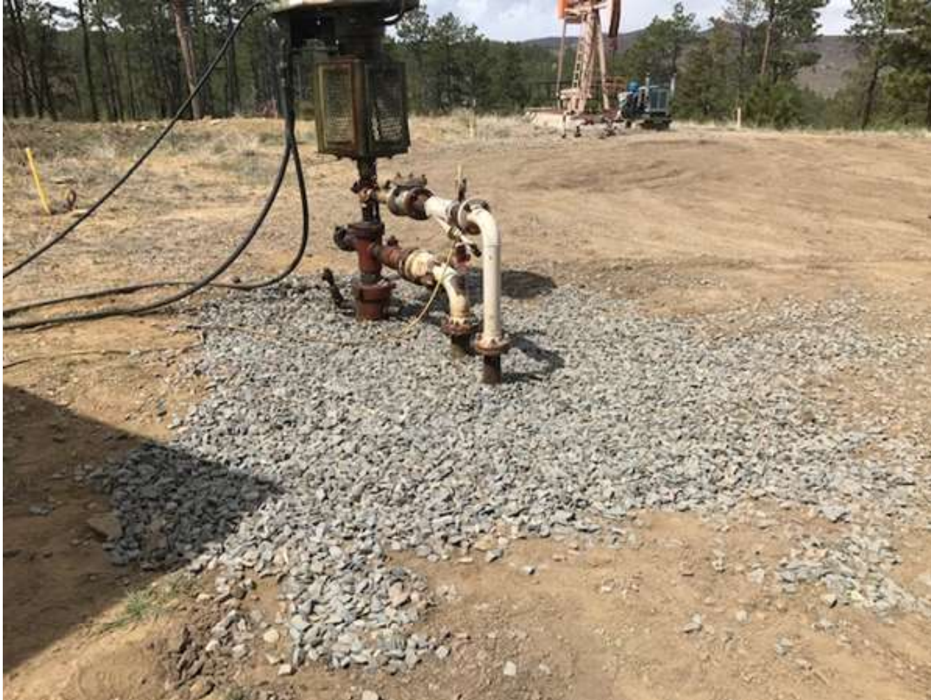
PHOTO 2: THE IMPACTED SOIL AROUND THE WELL HEAD AND ENGINE SKID WAS REMOVED FROM THE LOCATION.
