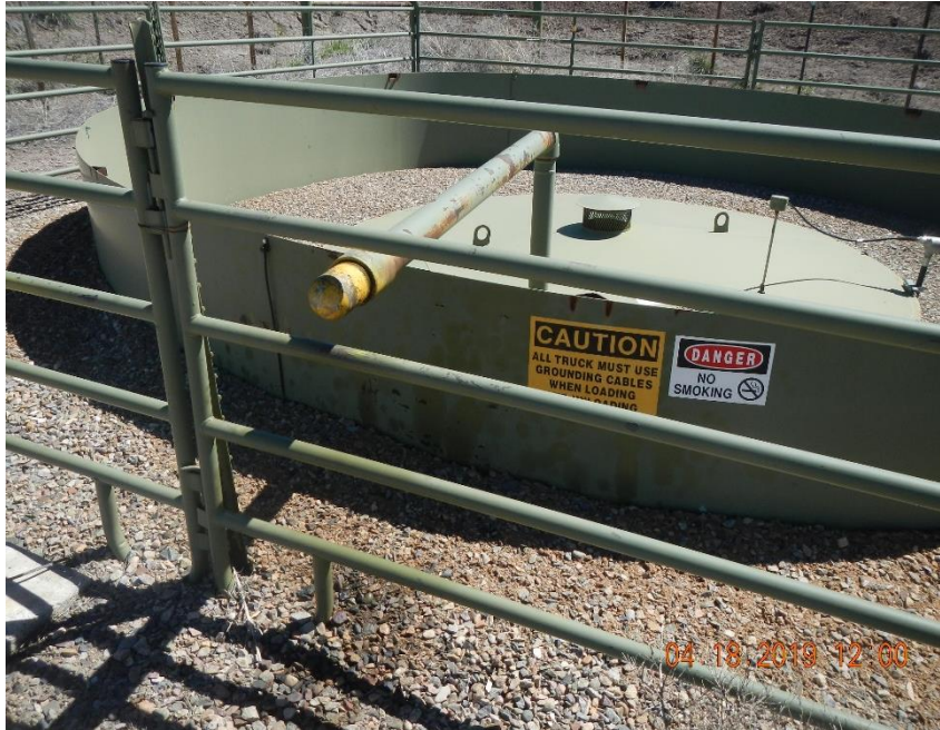
Stained gravel beneath truck load out valve for PBV.
