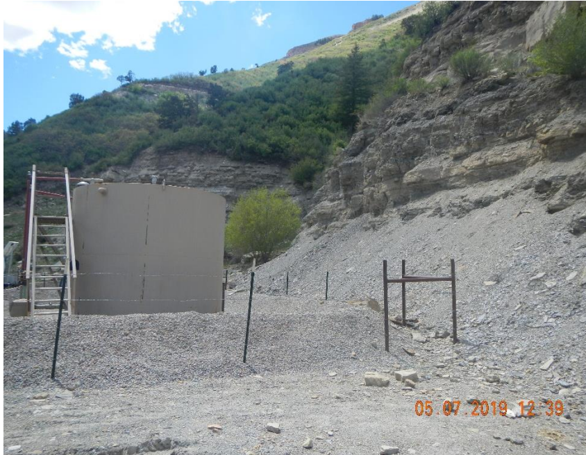
Photo 5 Shale, rock and sediment sloughing of cut slope against tank berm.
