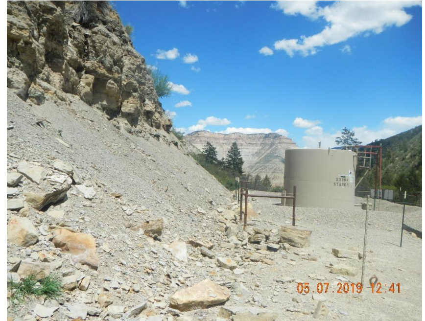
Photo 6 Shale, rock and sediment sloughing of cut slope against tank berm.
