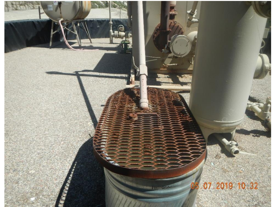
Photo 4 Secondary containment is full of fluid.
