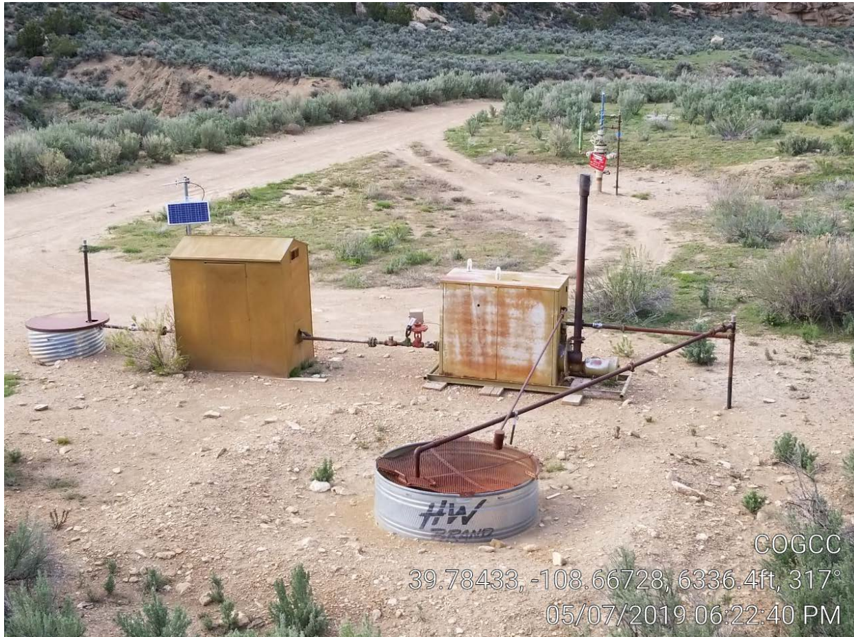
Photo 1. Location looking northwest.
