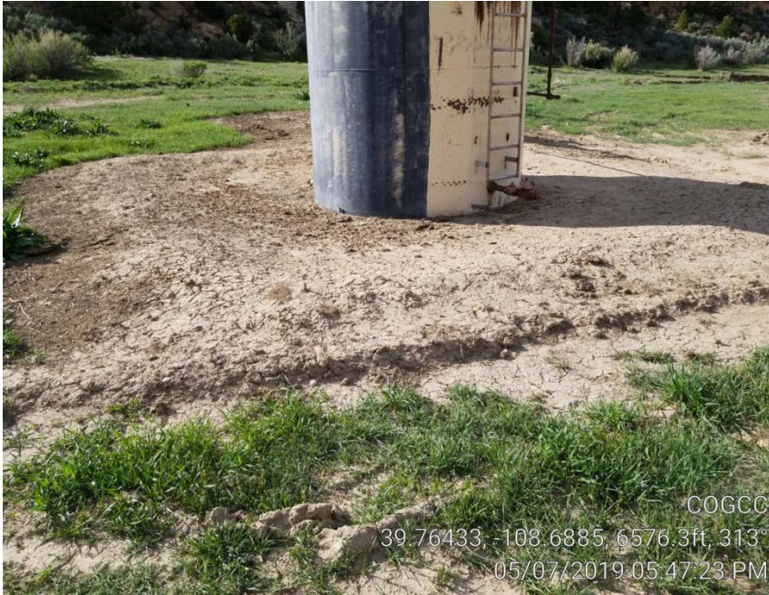
Photo 2. Inadequate tank berm.
