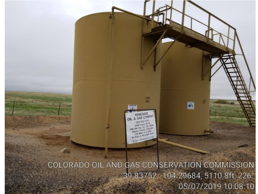
Pic 2 no cap on load line
