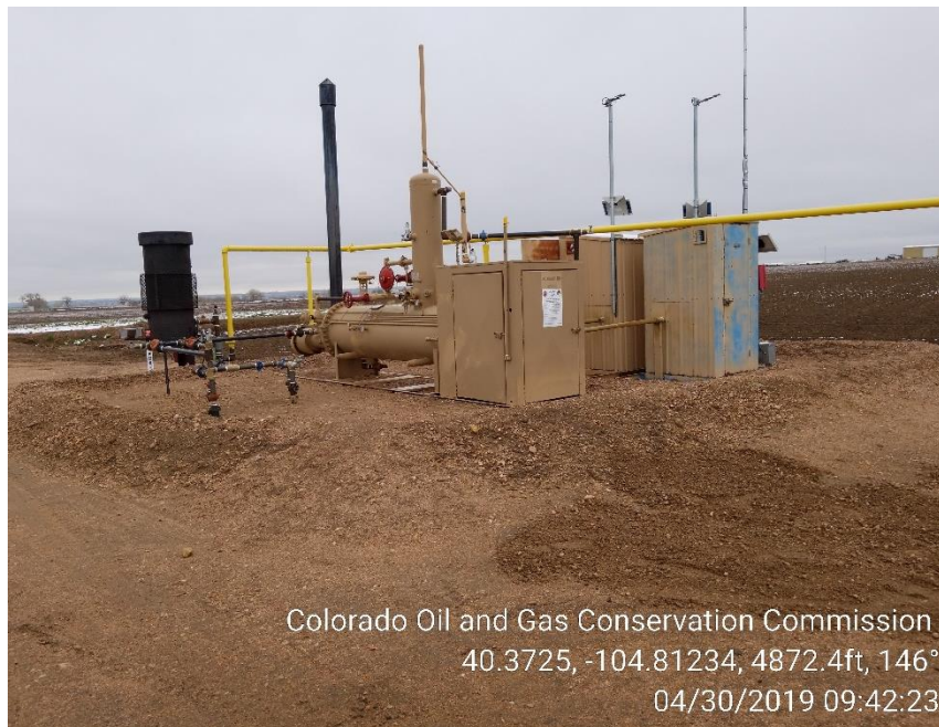
Photo 1 – Old separator has been replaced
