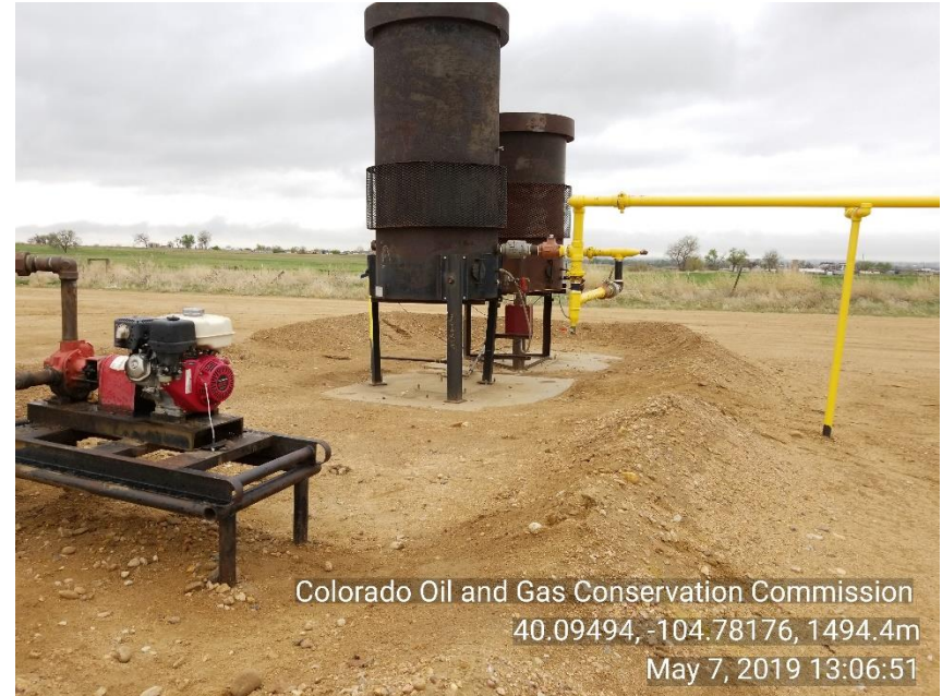
Photo 4 Stained soil under recir pump appears to be removed and 1 ECD running and other shut in.
