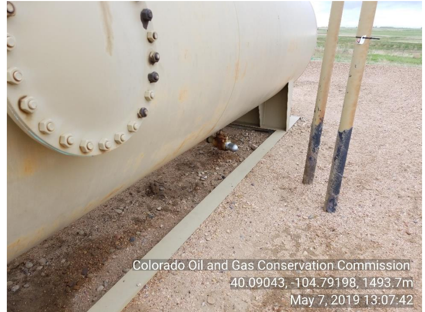
Photo 6 bull plug installed.
