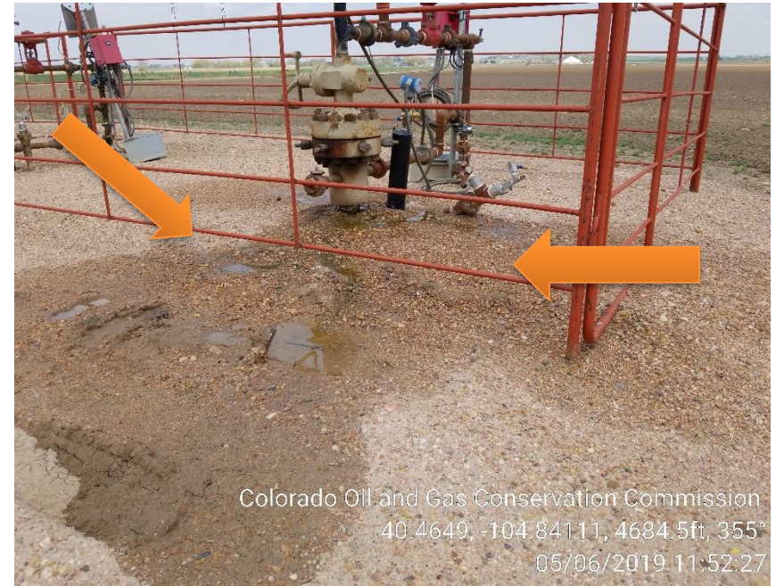
Photo 2 – Area of non know substance around wellhead.
