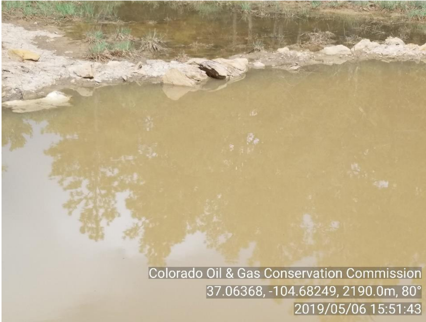
PHOTO 3: PIT IS PULL ALMOST RUNNING OVER THE EDGE. THERE IS NO 2' FREEBOARD MARKER. Lower fluid level so at least two feet of freeboard exists per Rule 902.b. INSTALL FREEBOARD MARKER.
