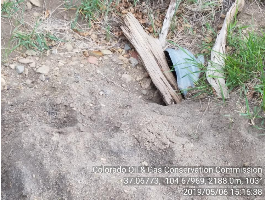
PHOTO 3: CULVER ON ROW NORTHWEST OF LOCATION IS PLUGGED. Install or repair required BMPs per Rule 1002.f.
