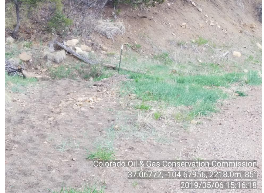
PHOTO 4: SEDIMENT HAS FILLED STORMWATER DRAIN ON UPSLOPE SIDE OF PLUGGED CULVERT
