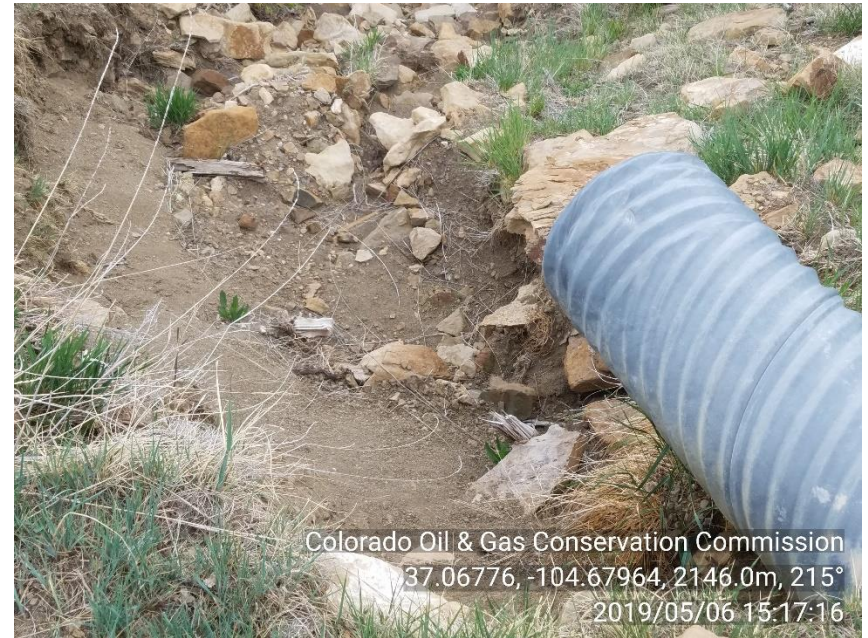
PHOTO 6: STORMWATER EROSION AROUND CULVERT OUTLET. Install or repair required BMPs per Rule 1002.f.
