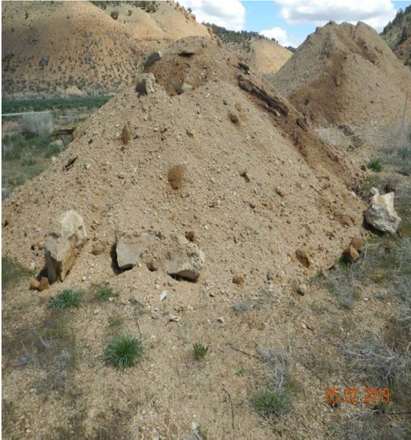
Photo#3: Stockpiles have no BMPs.
