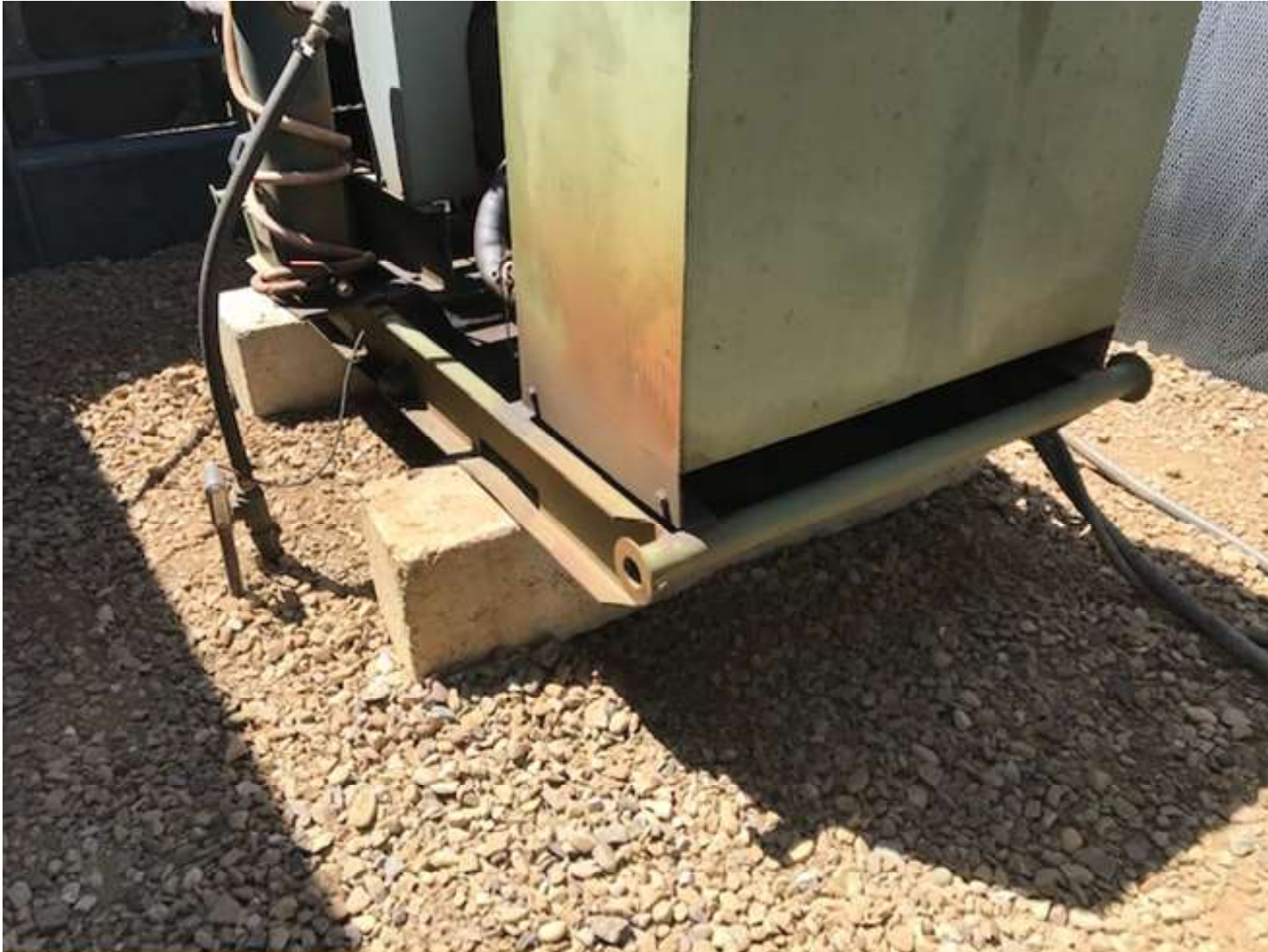
PHOTO 3: THE IMPACTED SOIL NEXT TO THE ENGINE SKID WAS REMOVED FROM THE LOCATION.
