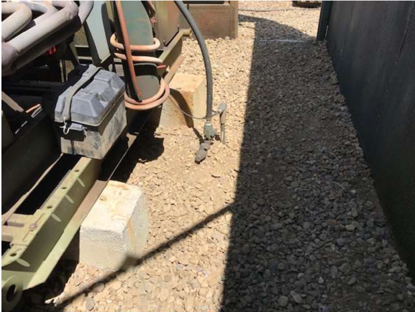
PHOTO 2: THE IMPACTED SOIL NEXT TO THE ENGINE SKID WAS REMOVED FROM THE LOCATION.
