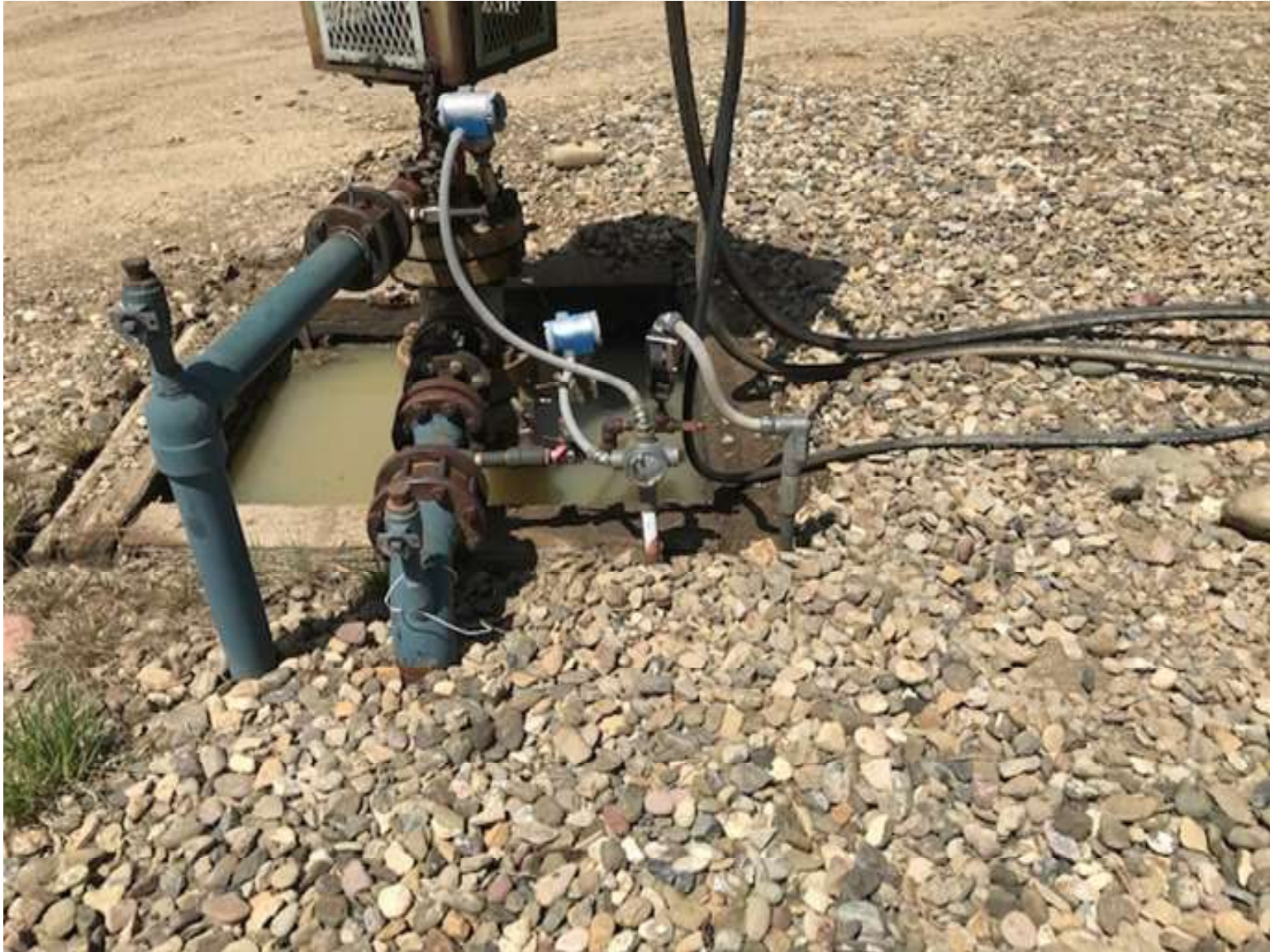
PHOTO 1: THE IMPACTED SOIL AROUND THE WELL HEAD WAS REMOVED FROM THE LOCATION.
