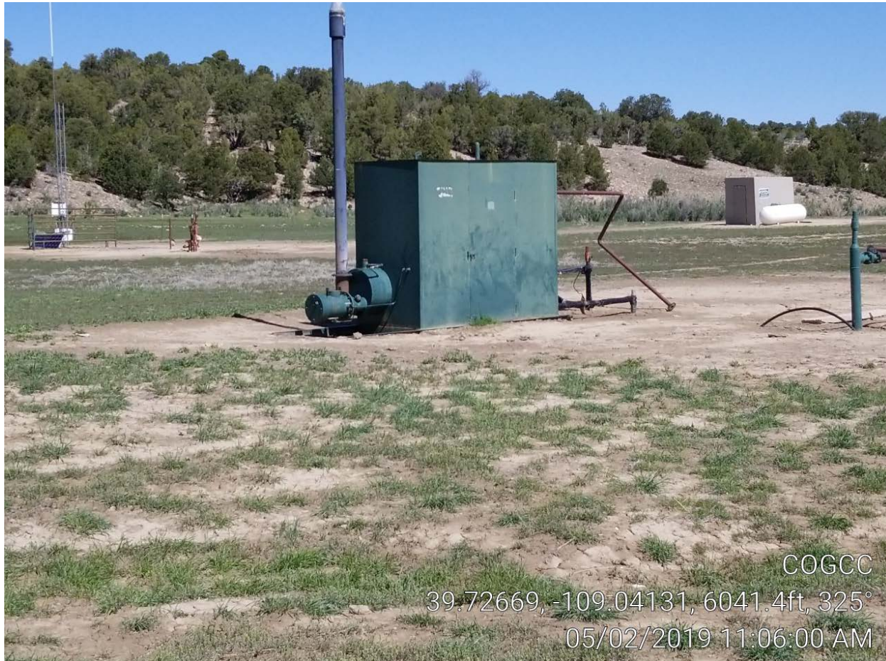
Photo 1. Location looking northwest.
