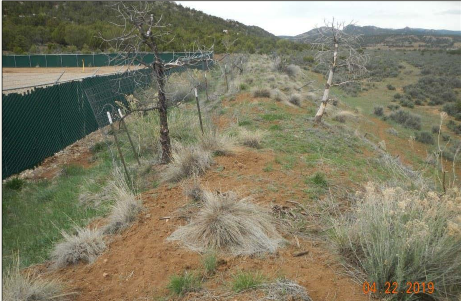
Photo 2. View of the eastern project area from the southeastern corner facing northward.
