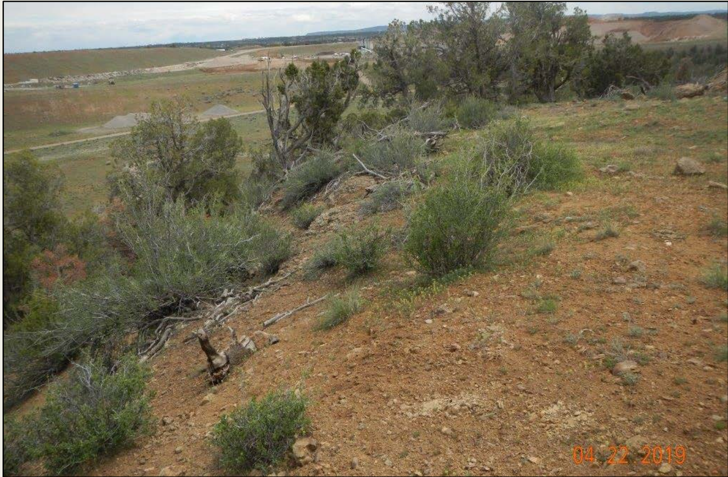
Photo 1. View of the western fill slope from the northeastern edge facing southeastward.
