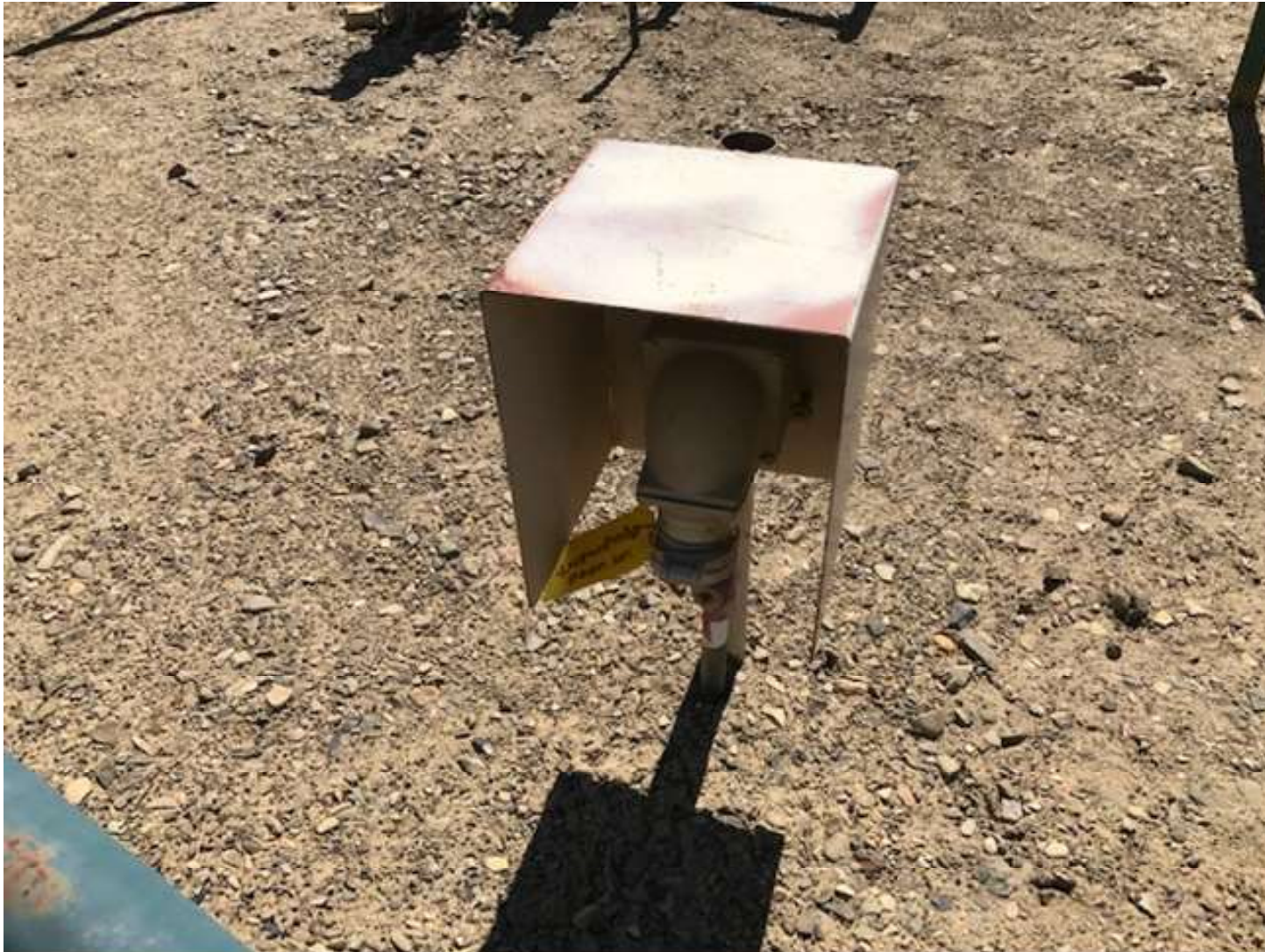
PHOTO 4: THIS IS AN ELECTRICAL BOX AND NOT A PIPELINE RISER, BUT WAS LABELED AS SUCH.
