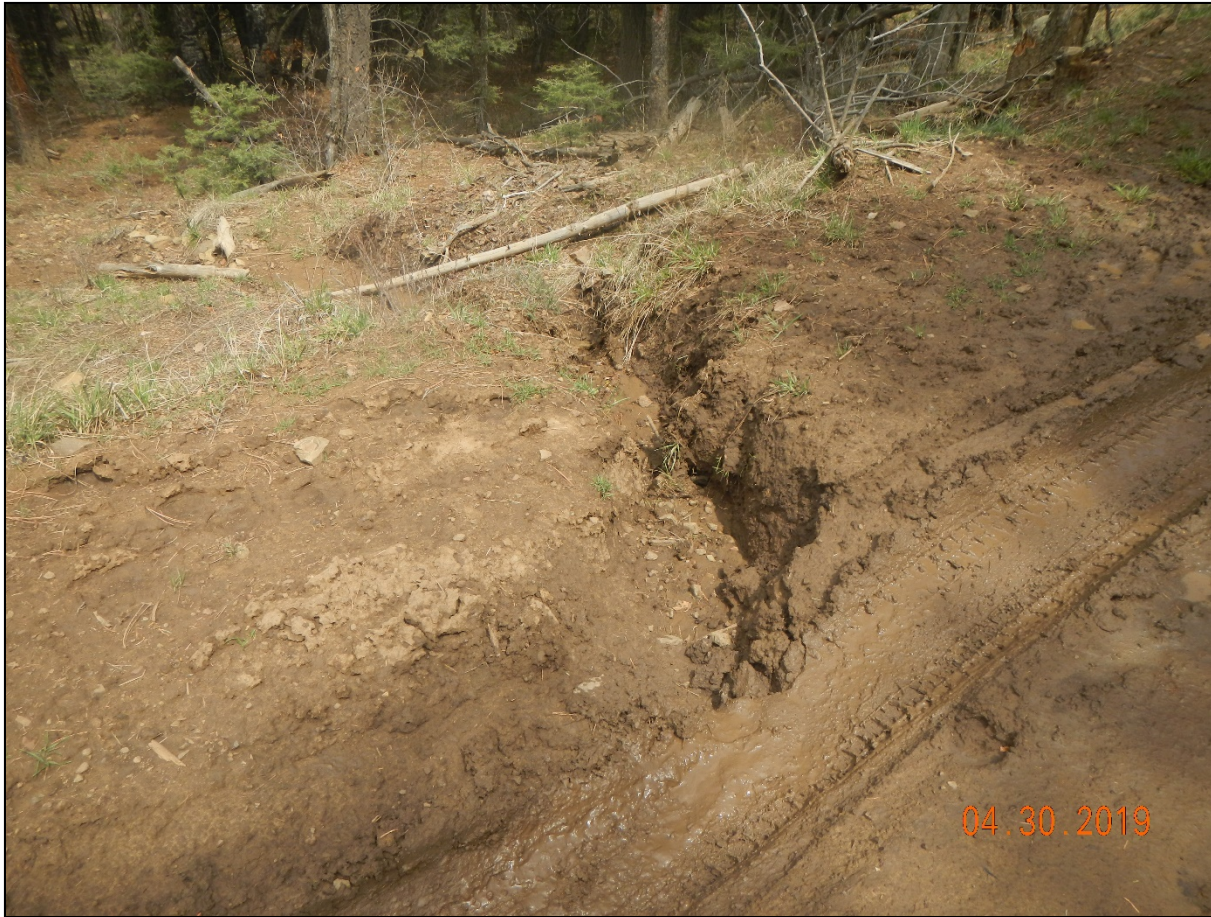
Photo 2. Stormwater flowing across the road in the previous photo is eroding the side of the road.
