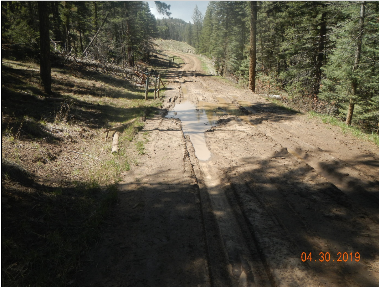
Photo 1. Facing west along the main access road. There is vehicle rutting along the road causing road damage. Stormwater is accumulating on the road.
