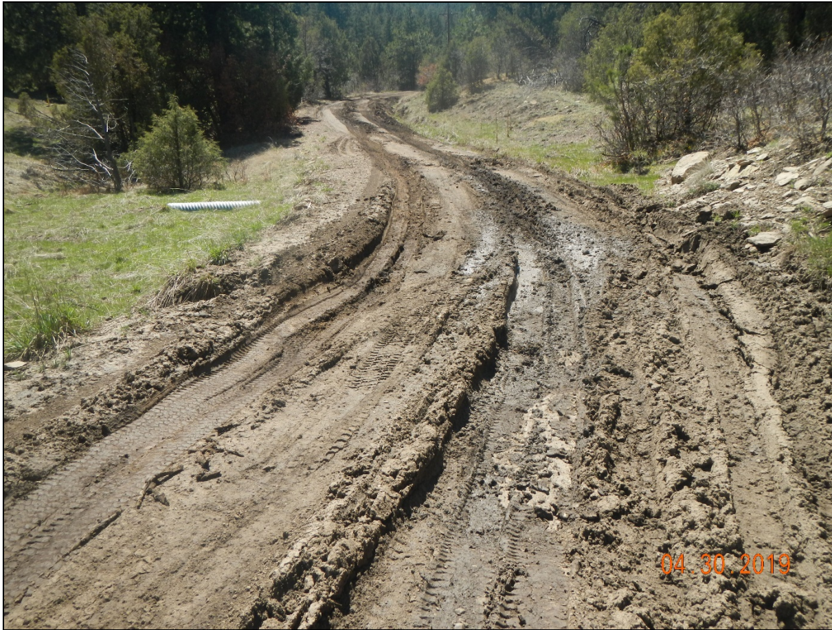
Photo 1. Facing west along the main access road. There is vehicle rutting along the road causing widening of the road.
