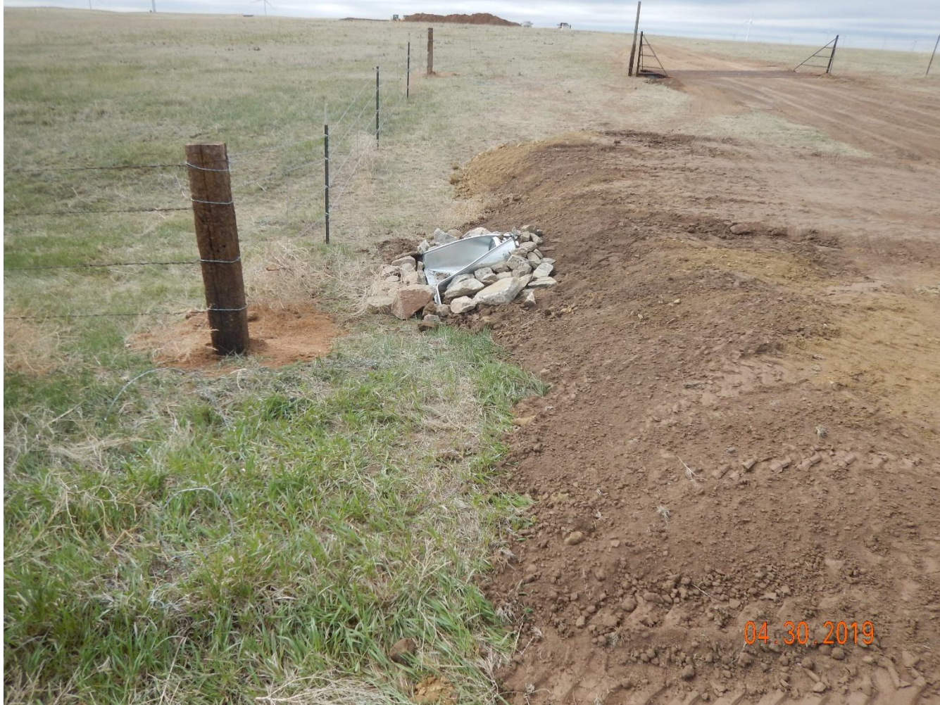
Photo 4: Photo taken from access road entrance. Photo shows culvert installed with inlet/outlet armoring.
