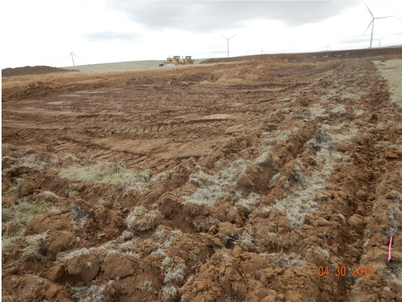
Photo 2: Photo taken from the northwest corner of the location, facing south. Photo shows construction activities in process. Photo also shows operator has installed surface roughening along perimeter of the location. .
