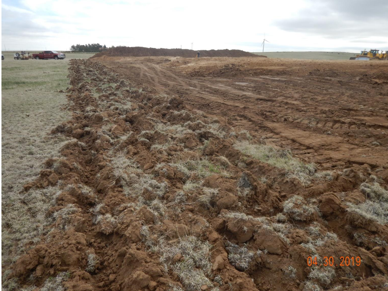
Photo 1: Photo taken from the northwest corner of the location, facing east. Photo shows construction activities in process. Photo also shows operator has installed surface roughening along perimeter of the location.
