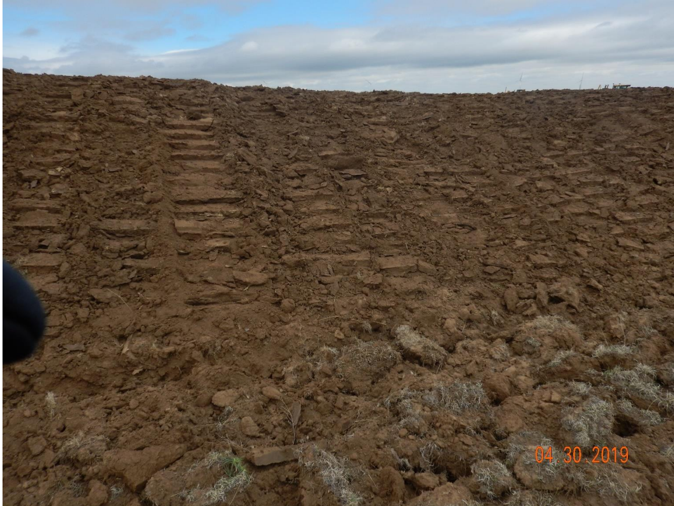
Photo 3: Photo taken from the soil stockpile on the south end of the location. Operator has implemented tracking to stabilize soil stockpiles.
